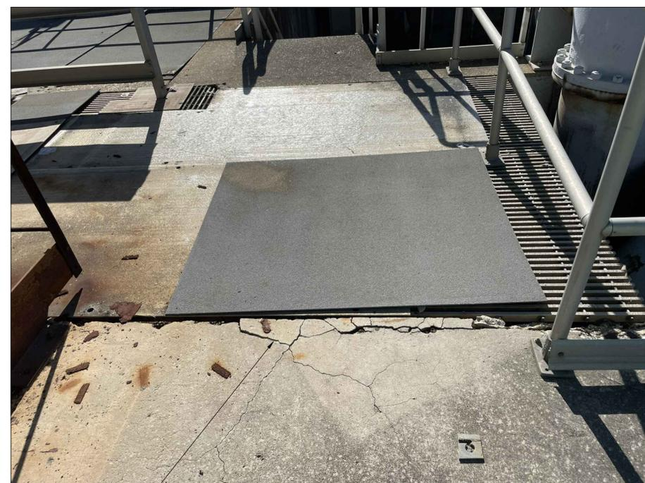
CRACKING AND SPALLING TO BE REPAIRED PER SHEET S-30-02
