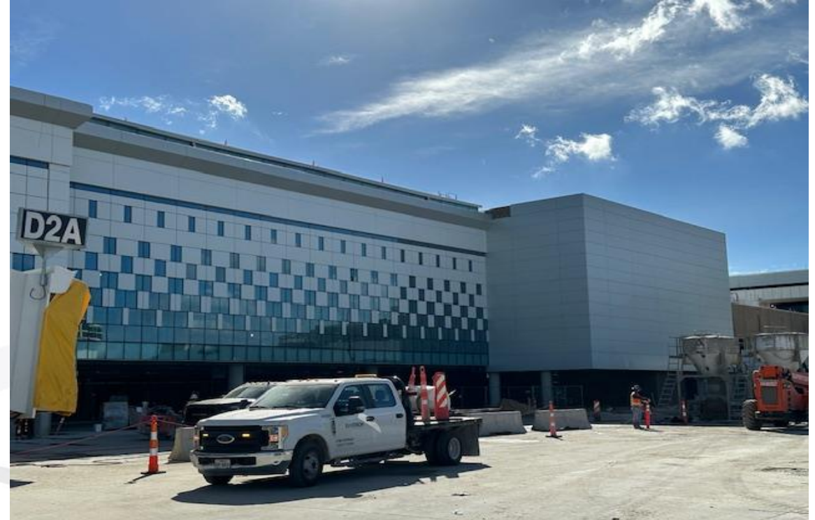
Feature wall - 13,600 sf (380 linear feet)
