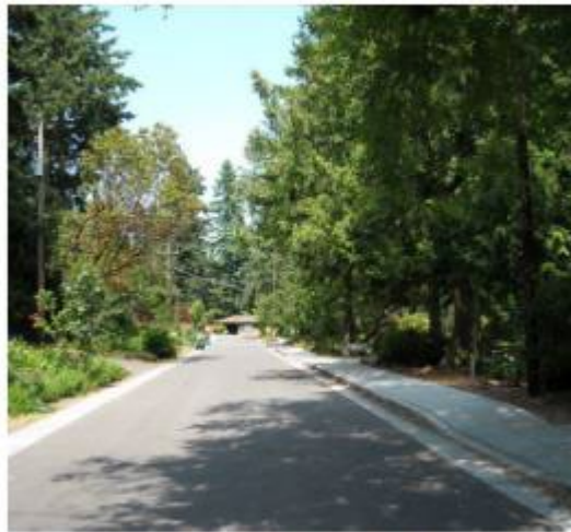
OD-2.3 Built example of regraded street with concrete sidewalk and a consolidated bioswale on one side of the street
