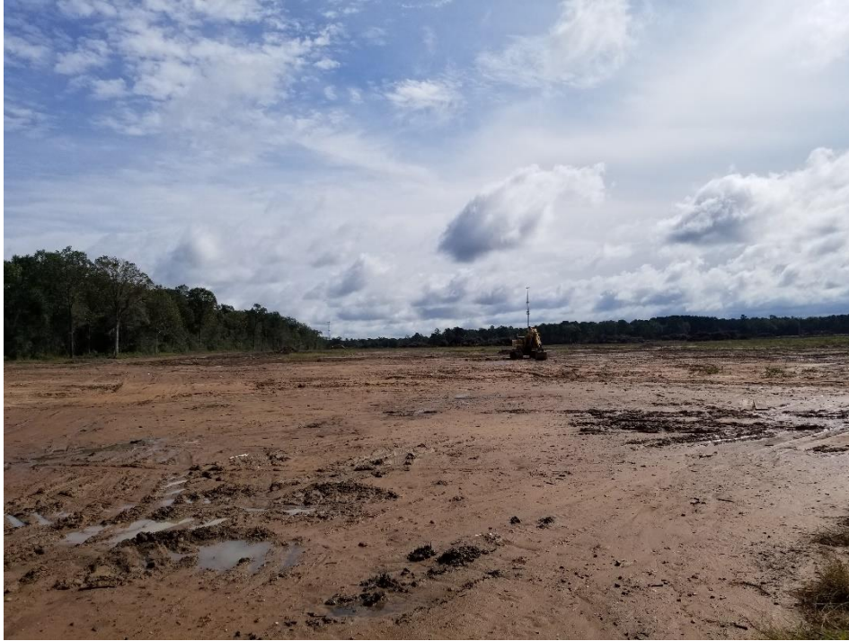
View from Construction Site on Webb Road Looking East
