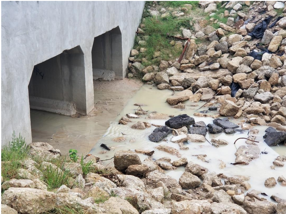
Close View of Box Culverts on Taylor Gulley
