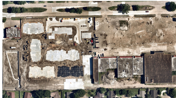
Construction of Edison Lofts, 2020
