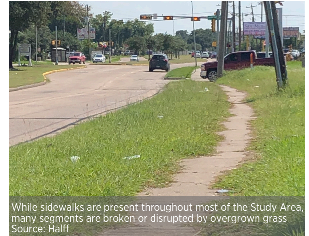
Discontinuous sidewalk segment along Fondren Rd. Source: Half
