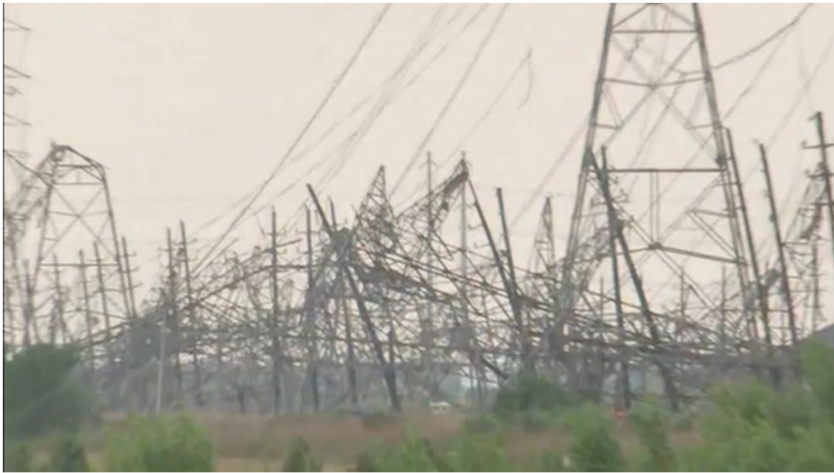
Figure 4: Infrastructure Damage – Destroyed Power Towers
