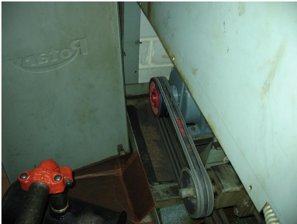
Photo 6: Photo of the reservoir closet for the elevator shown in photo #5. De minimis staining is visible under the equipment.
