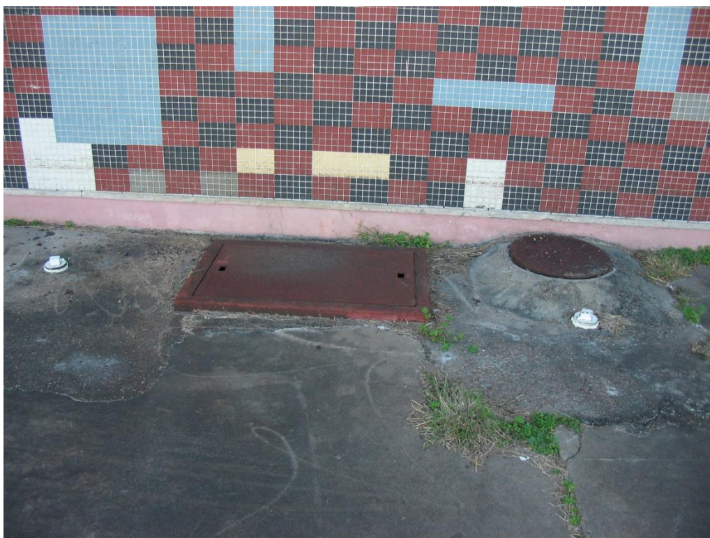
Photo 15: Photo view shows an active grease trap on the western exterior wall of the retail building.
