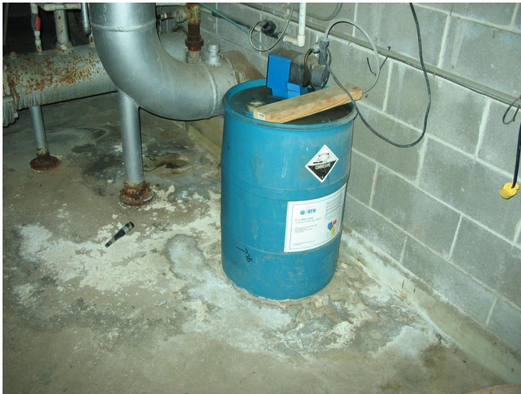
Photo 9: Photo view of drum containing C-1300 LPH, cooling water treatment chemicals showing corrosion stains on the floor of the penthouse.
