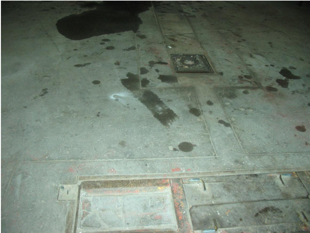
Photo 22: Hydraulic lift set in the ground inside the automotive garage.
