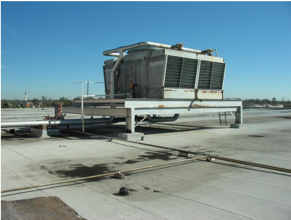
Photo 10: HVAC cooling tower on the roof of the retail building.
