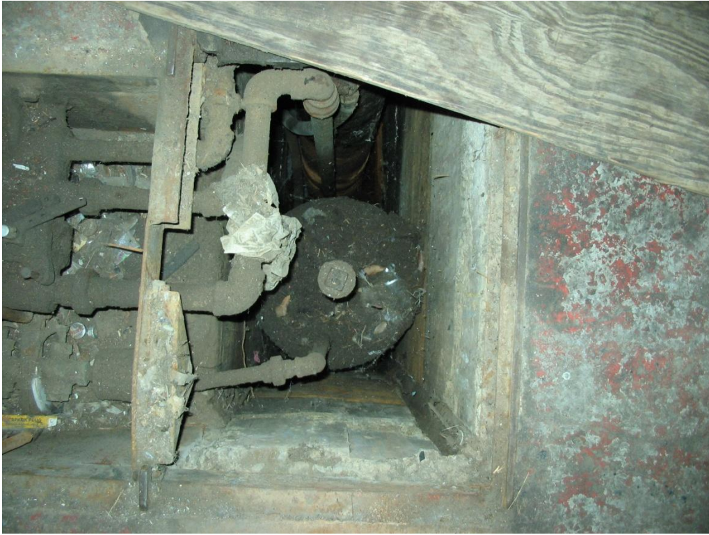
Photo 21: View of reservoir and equipment associated with one of at least eight hydraulic lifts set in the ground of the automotive garage.
