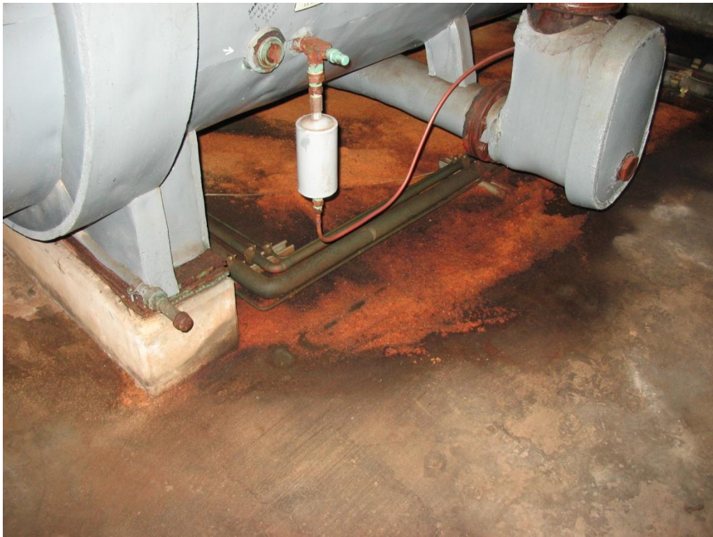
Photo 8: Staining under the chiller inside the mechanic penthouse and associated with the HVAC system.
