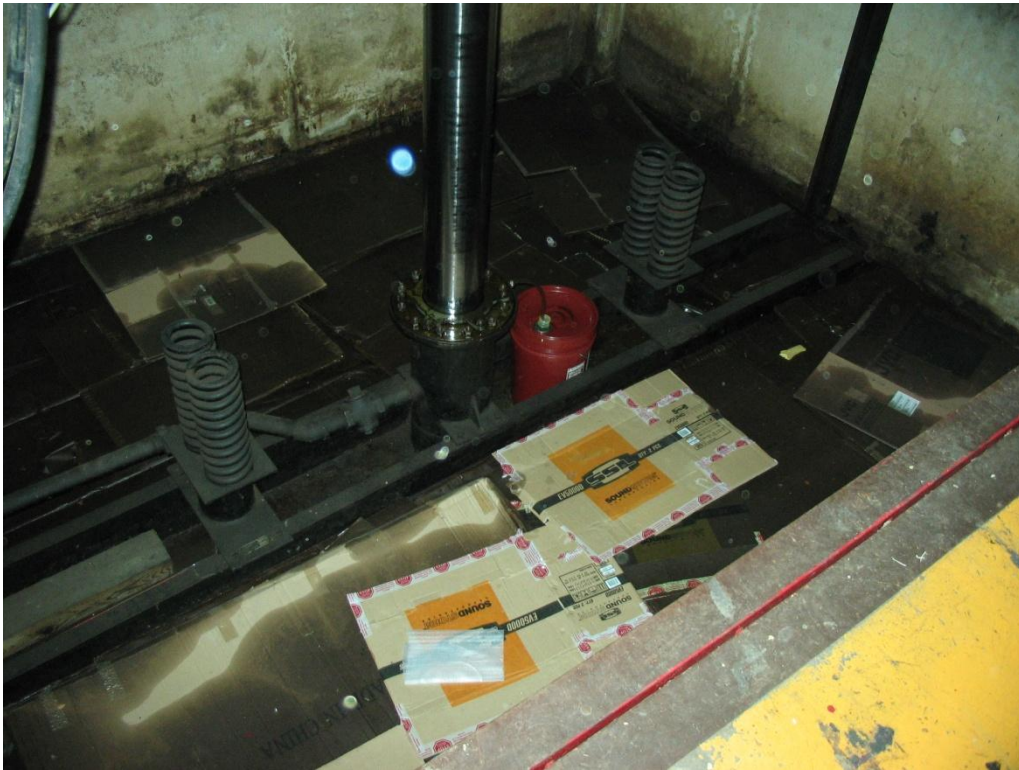
Photo 13: View of pit below the freight elevator near the southwest corner of the retail building. Excessive staining of hydraulic fluid was present within the pit and cardboard used to absorb the fluid prevented observation of the ground surface.
