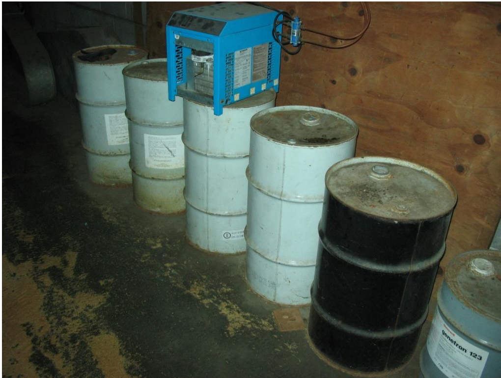
Photo 7: Drums containing water treatment chemicals for the cooling tower associated with the HVAC system, stored inside the mechanic penthouse.
