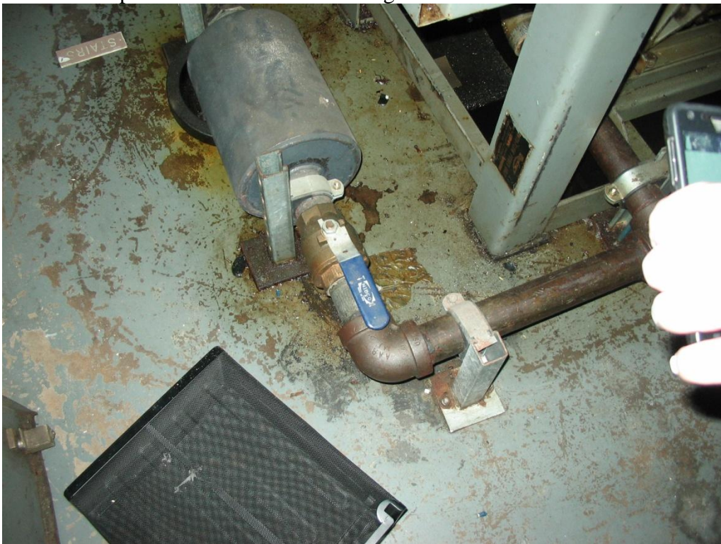
Photo 14: Photo of the reservoir closet for the freight elevator shown in photo #13. De minimis staining is visible under the equipment.
