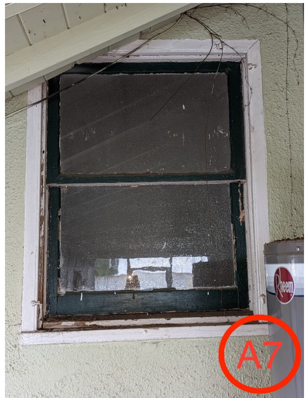
Figure 15 - Window on Rear Porch
