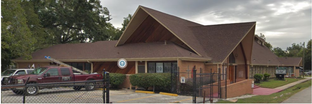
WEST FACE ALONG LUCINDA STREET BY GOOGLE STREET VIEW
