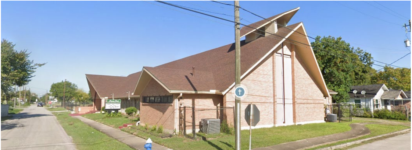
EAST FACE ALONG MILBY STREET BY GOOGLE STREET VIEW
