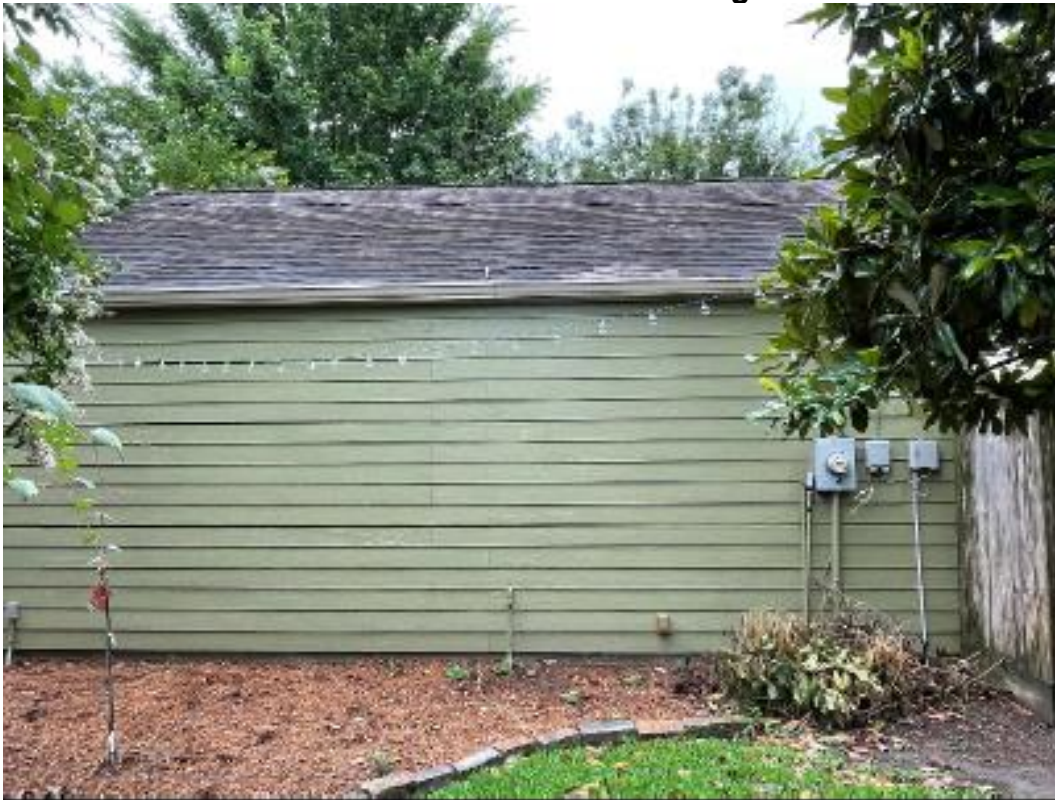
North side of Detached Garage
