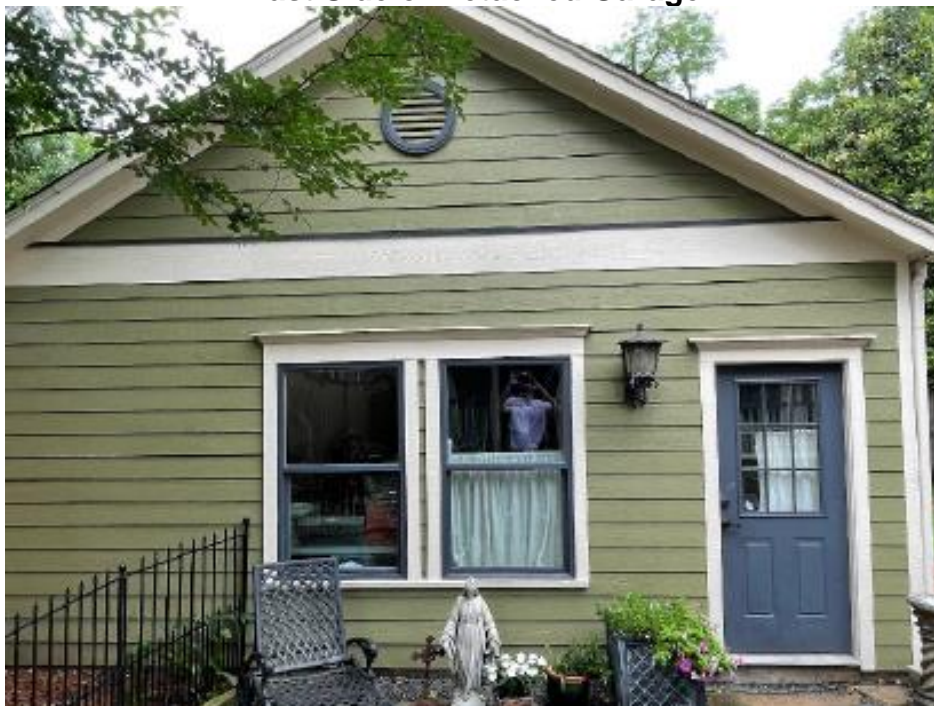
East Side of Detached Garage
