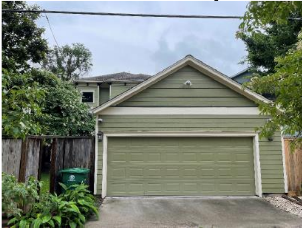
West side of Detached Garage
