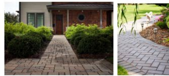
FRONT WALKWAY: material and pattern to be coordinated with low threshold wall Pictured: Concrete pavers in ashlar pattern and traditional bricks in herringbone with a soldier course.
