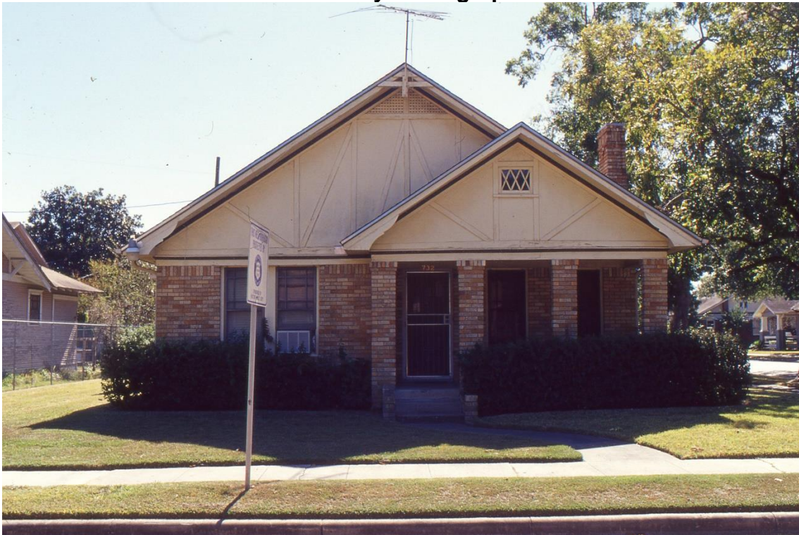
732 W Cottage St: Main structure
