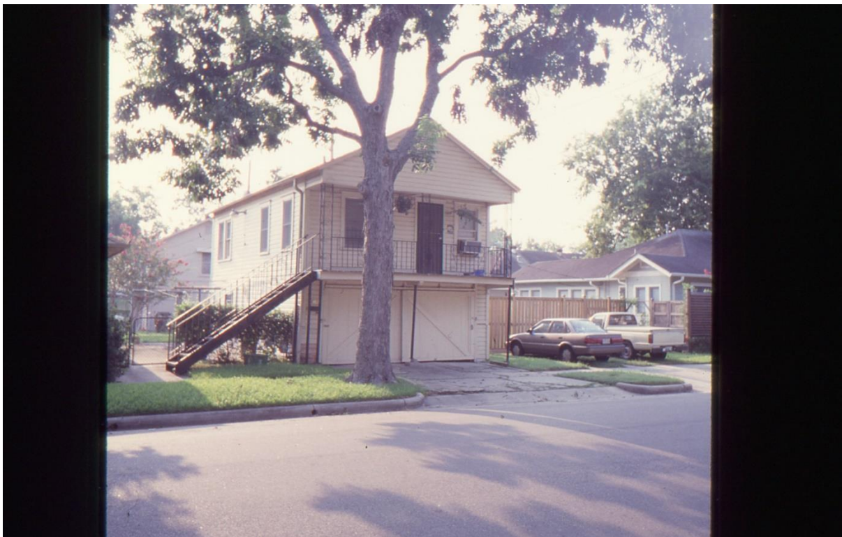
3810 Watson: detached garage of 732 W Cottage
