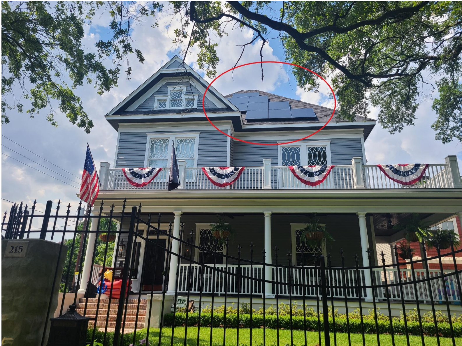
Front of house (facing south)
