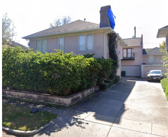
607 Marshall St – Contributing – 2014 (across street)
