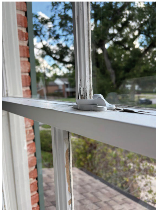
Bedroom window (EX23) – moisture damage from leaking at interior sash
