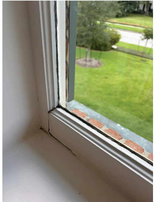
Laundry window (EX20) – moisture damage and wood rot from leaking at interior sash
