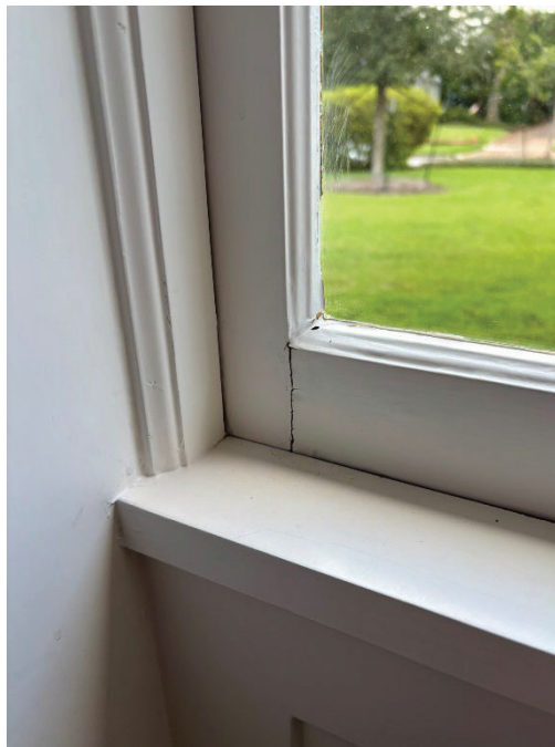
Living Room window (EX01) – moisture damage at interior sash
