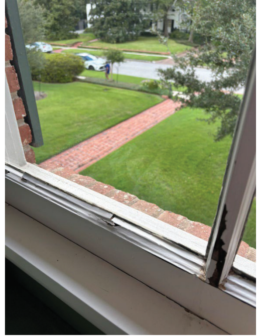
Bedroom window (EX22) – moisture damage and wood rot at interior sash
