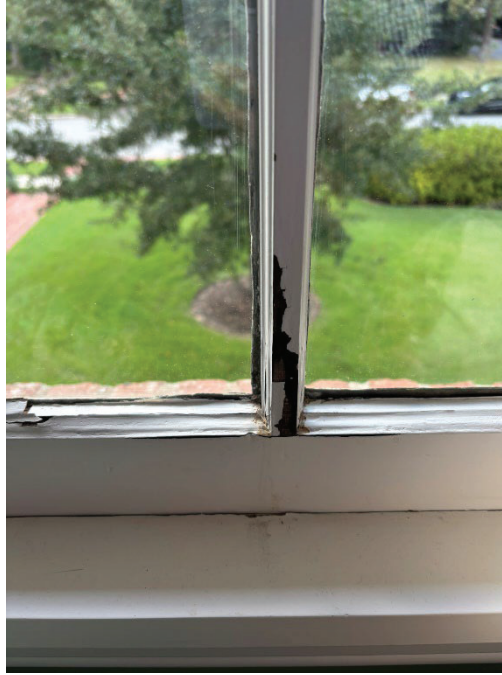
Bedroom window (EX22) – moisture damage and wood rot at interior sash
