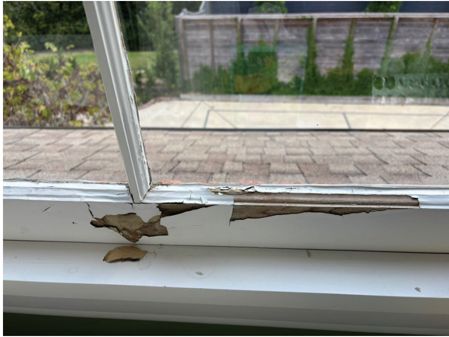
Bedroom window (EX23) – moisture damage from leaking at interior sash
