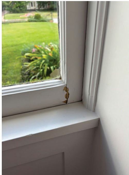
Living Room window (EX02) – moisture damage at interior sash
