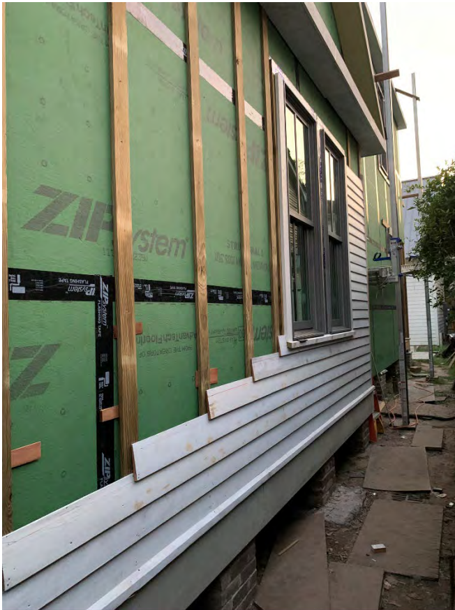
Figure 1 - Proposed Siding Replacement Method
