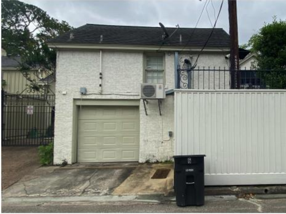
EXISTING WEST FACADE
