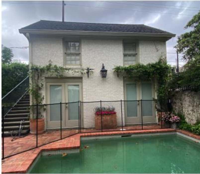
EXISTING EAST FACADE
