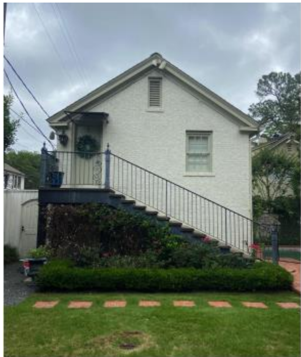
EXISTING SOUTH FACADE
