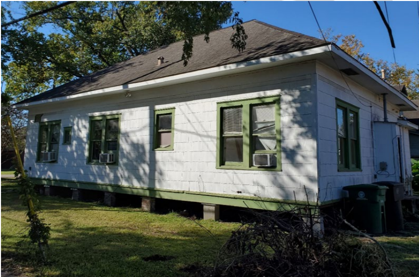
East - existing conditions
