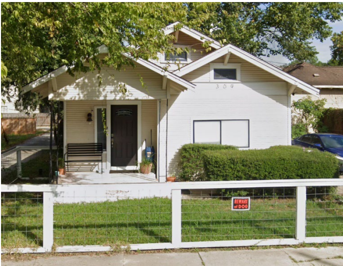
Figure 1-309 E 5th St, next door neighbor
