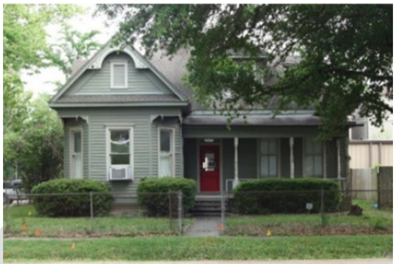
Figure 2-301 E 5th St, next door neighbor
