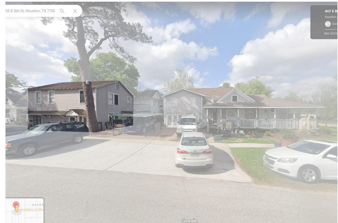
405 East 8th Street Non-Contributing Built 1940 Garage Apartment Two story volume with gable roof with similar fenestration and attic vent to 540 Cortlandt. Similar relationship of garage to main house adjacent.
