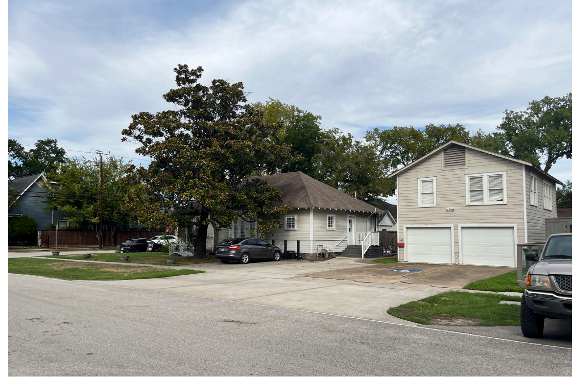
Photo 03 540 Cortlandt West/ South Elevation
