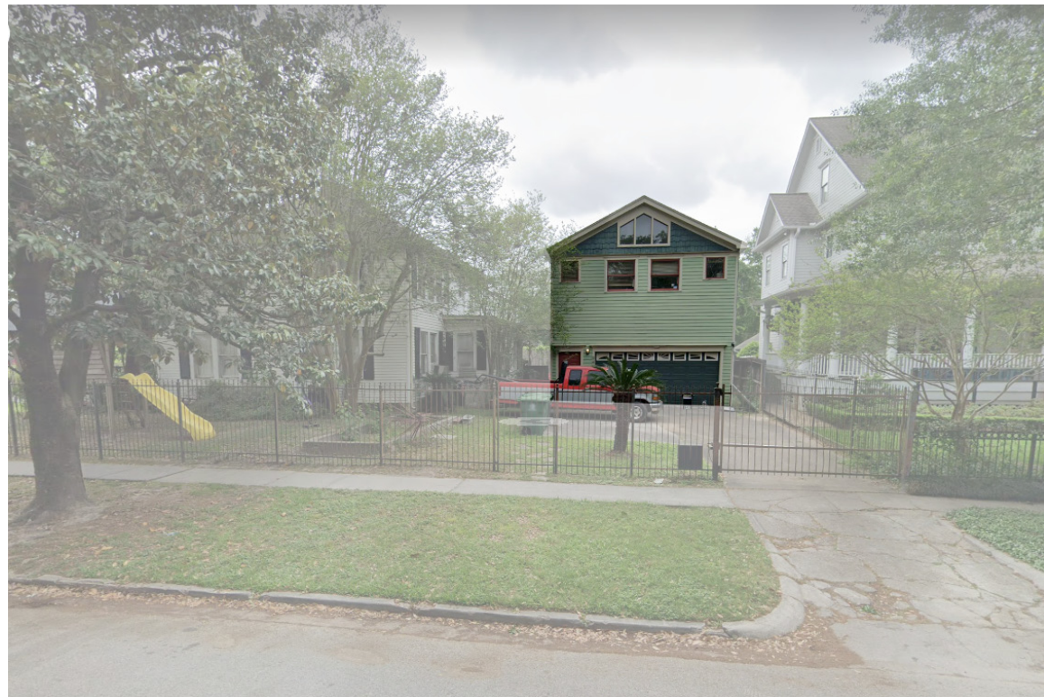
940 Harvard Street Non-Contributing Built 2000 Garage Apartment Similar two story Garage structure with gable roof at rear. Fen- estration facing street similar in style to 540 Cortlandt.
