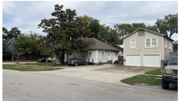
Photo 03 540 Cortlandt West/ South Elevation
