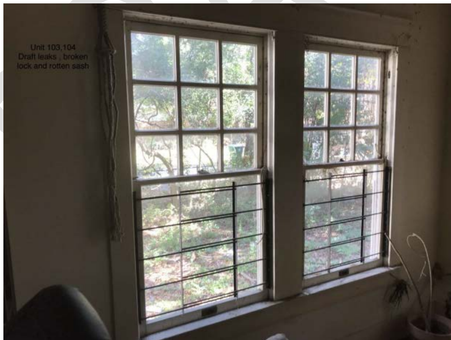
Figure 4—Interior view of windows 103 and 104
