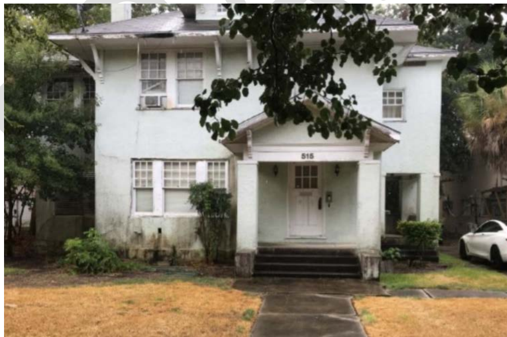
Figure 2-Two of Three Windows to be replaced
