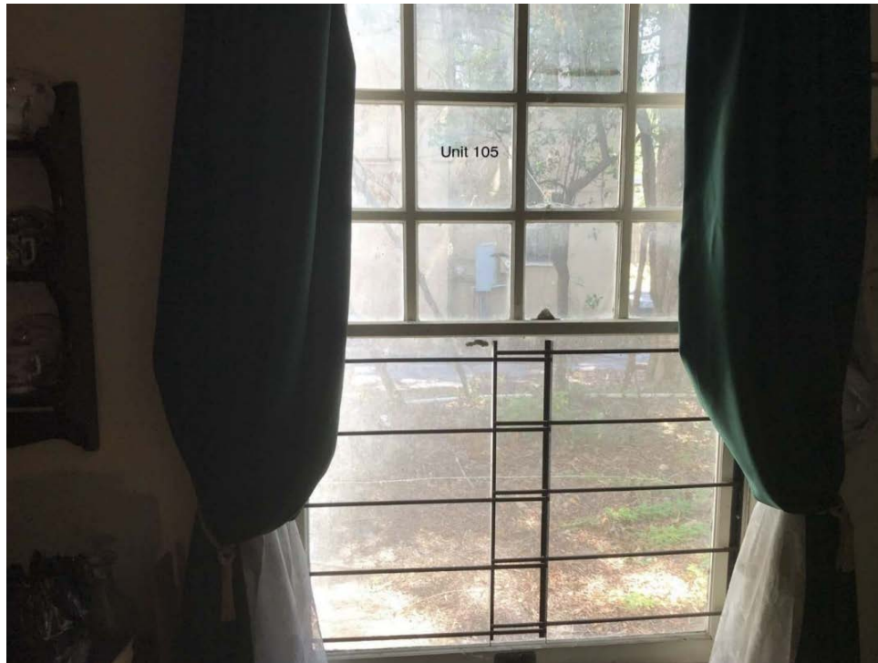
Figure 4-Interior view of window 105
