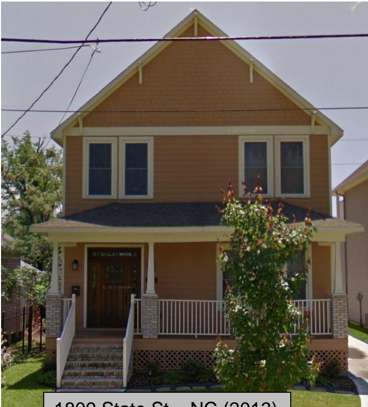
1809 State St – NC (2013) Max ridge height at 33' FFE at 2' 8:12 roof pitch Front Setback 20' Total sq. ft. 2,737
