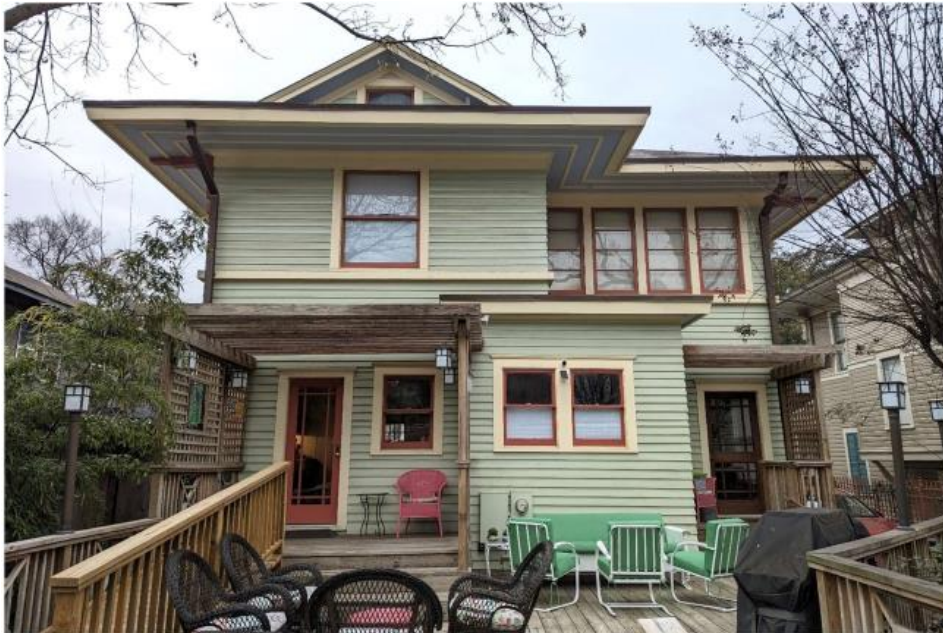
West (rear) elevation, January 2024. Downstairs non-original porch, pergola, and rear door to be removed are visible at far right. Upstairs rear window(s) to be removed (one or two, depending on size of elevator equipment) are visible at far right.
