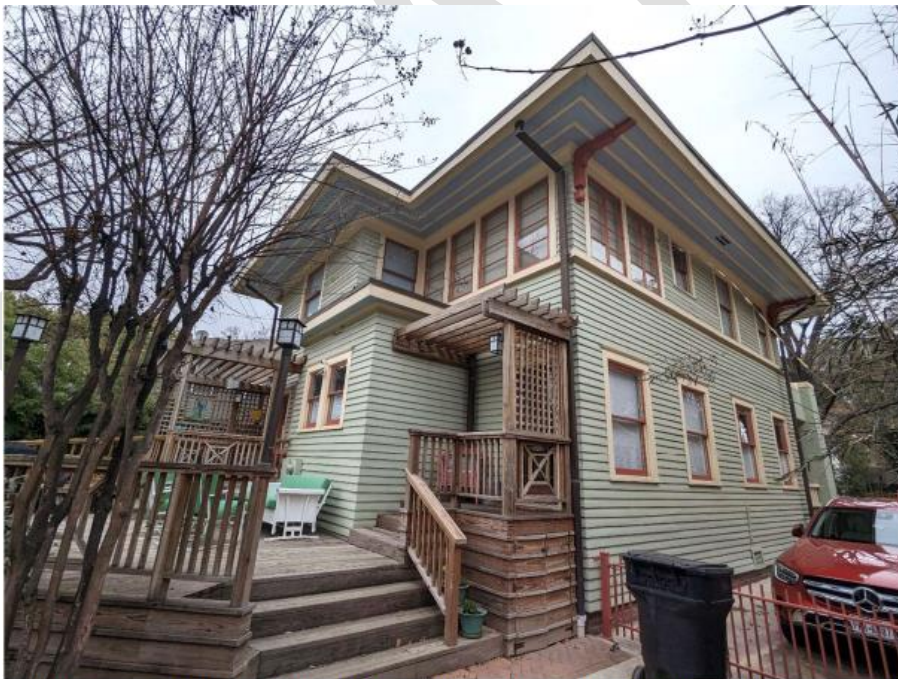
Southwest corner, January 2024. Downstairs non-original porch and pergola to be removed are visible at center. Upstairs rear window(s) to be removed (one or two, depending on size of elevator equipment) are visible above.
