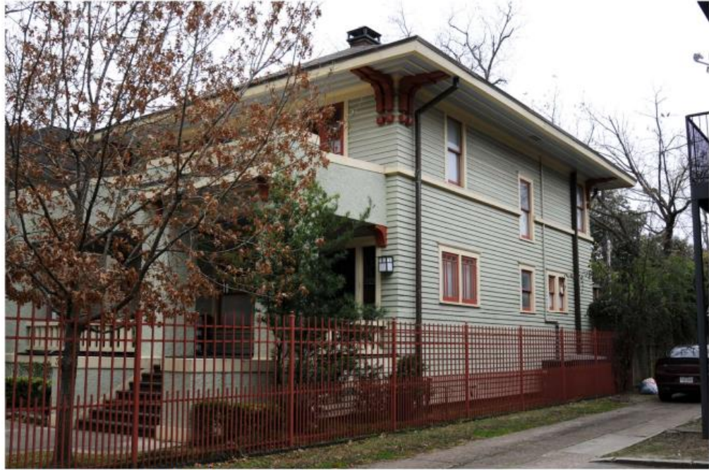
Northwest corner, January 2024
