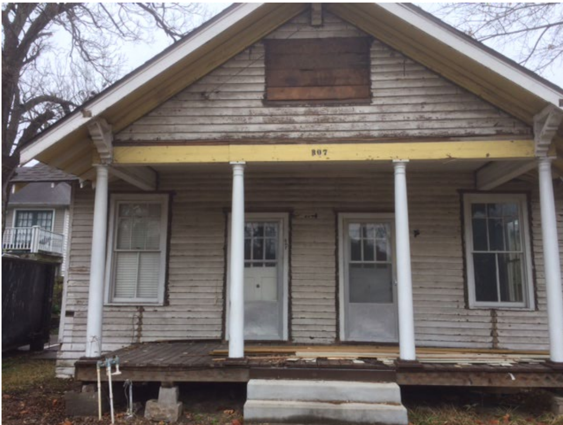
Figure 1 - 2018 After Synthetic Siding Removed
