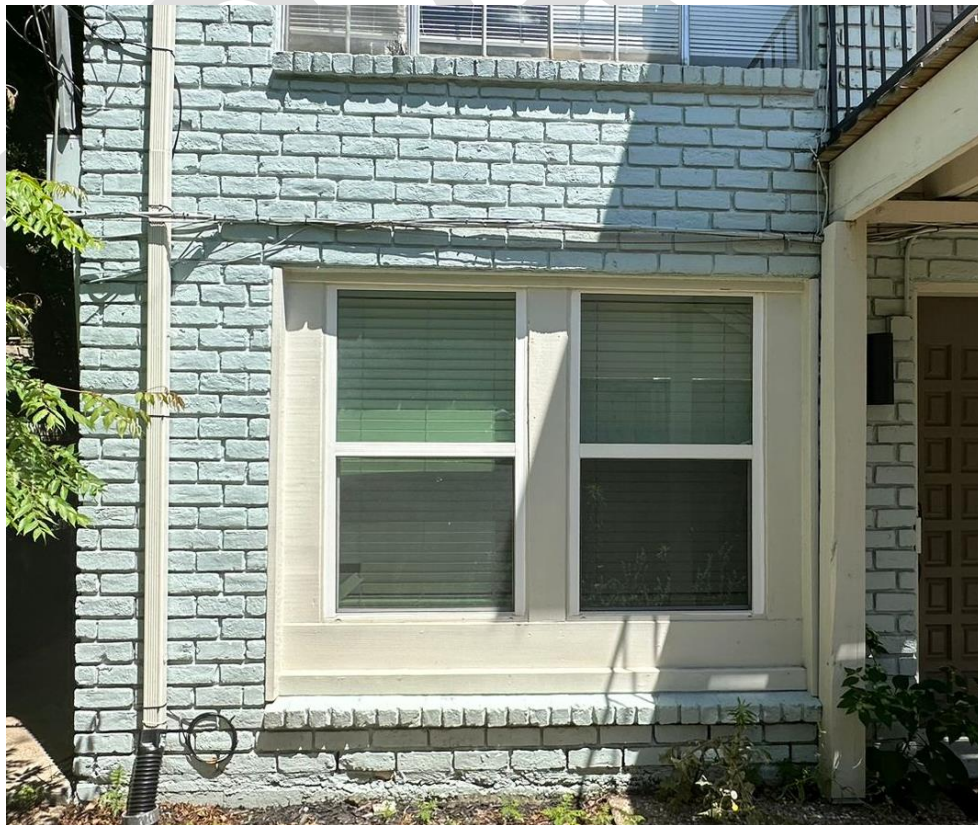
Window Example After Replacement
