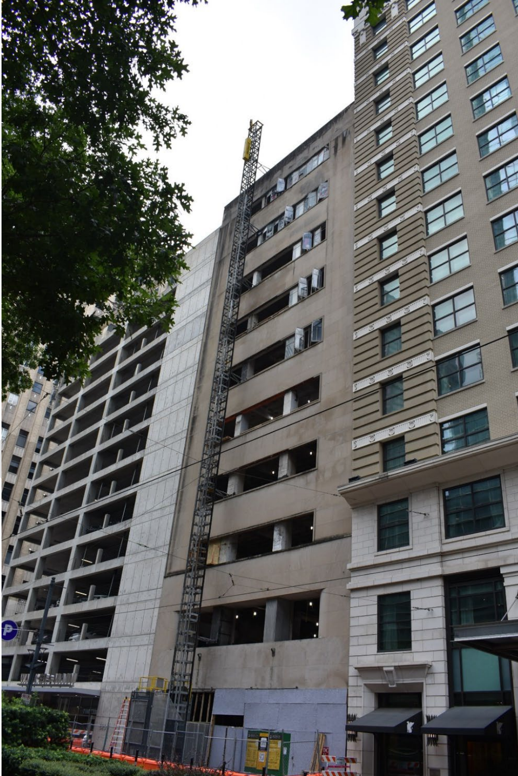
Photo 2: Oblique view of the east (front) elevation facing Main Street. Camera facing west. Photo by applicant, 2024.
