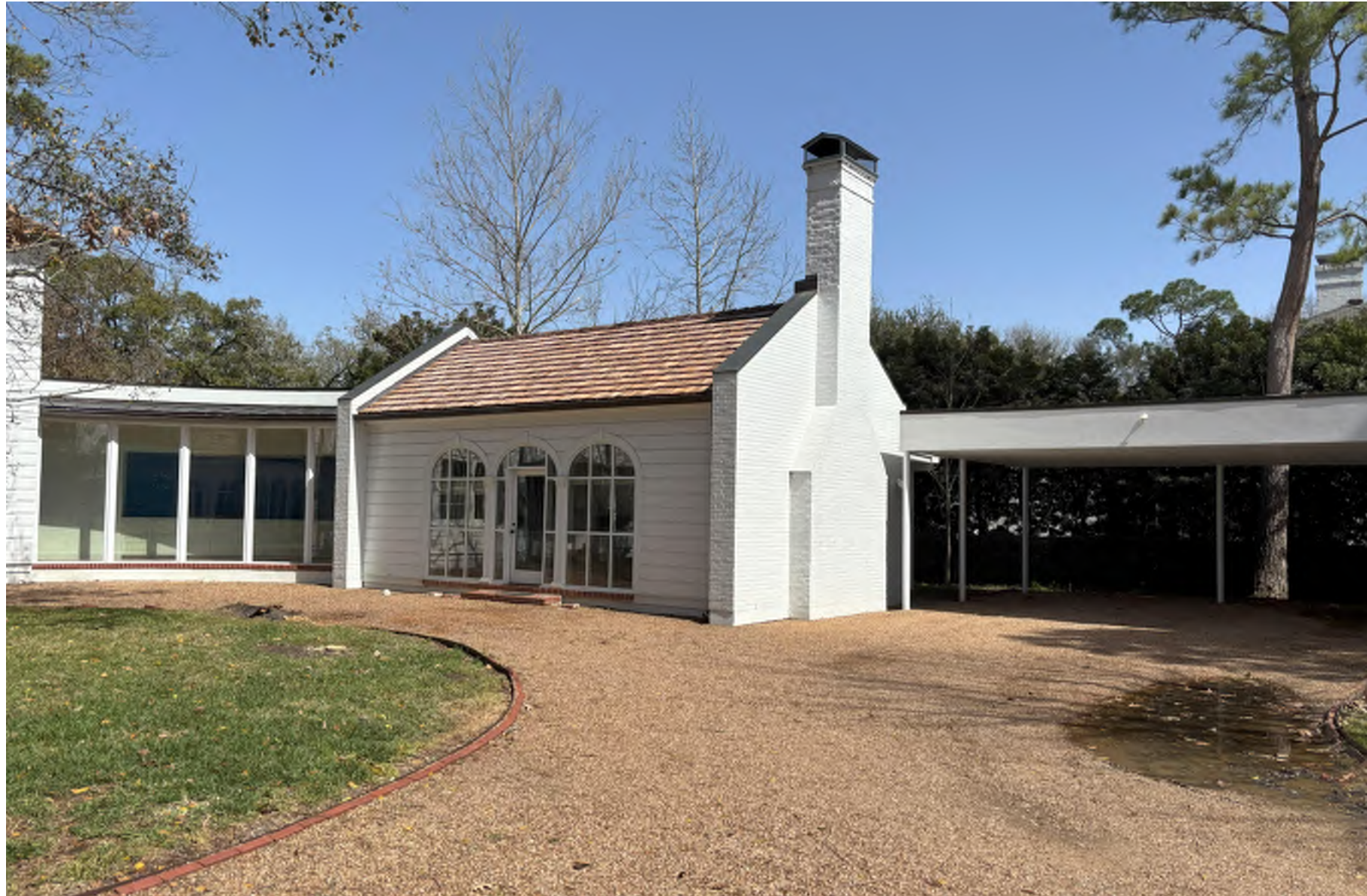
IMAGE 10. View looking northeast - 2002 renovation: addition of painted brick walls to the kitchen building, original kitchen windows ( Image 3 ) removed and replaced with mill work that matches the screened porch windows ( Image 8 ), original arcade walkway enclosure ( Image 4 ) demolished and replaced with floor to ceiling glass windows. - Current
