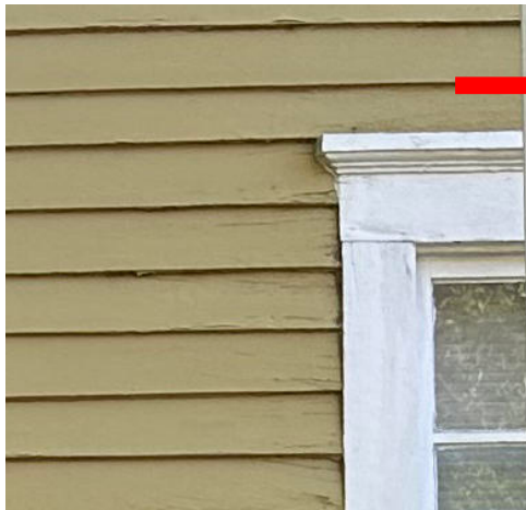
Existing Wood Lap Siding & Trim Lap Siding: 4 1/2" Exposure Height
