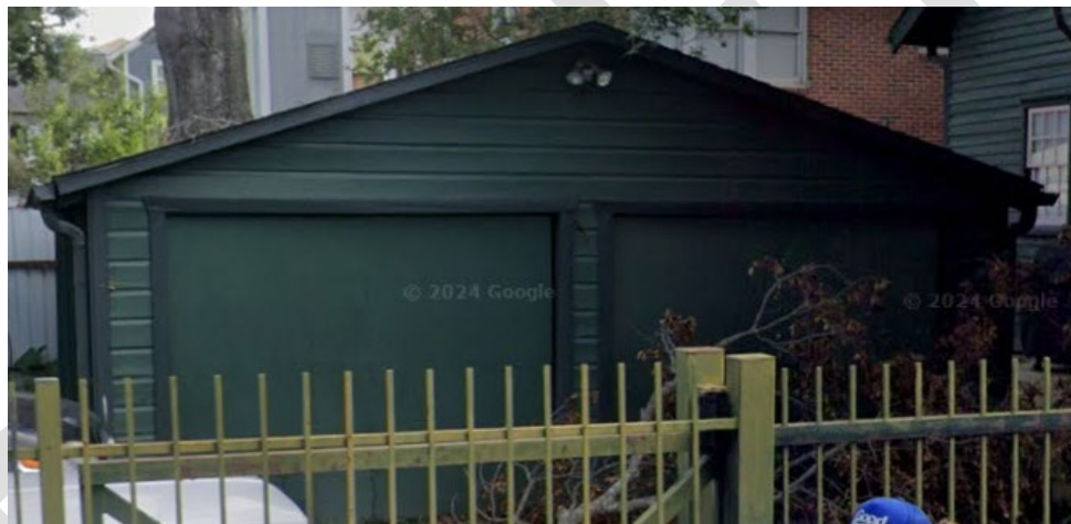
NON-CONTRIBUTING GARAGE (SUBJECT OF COA)
