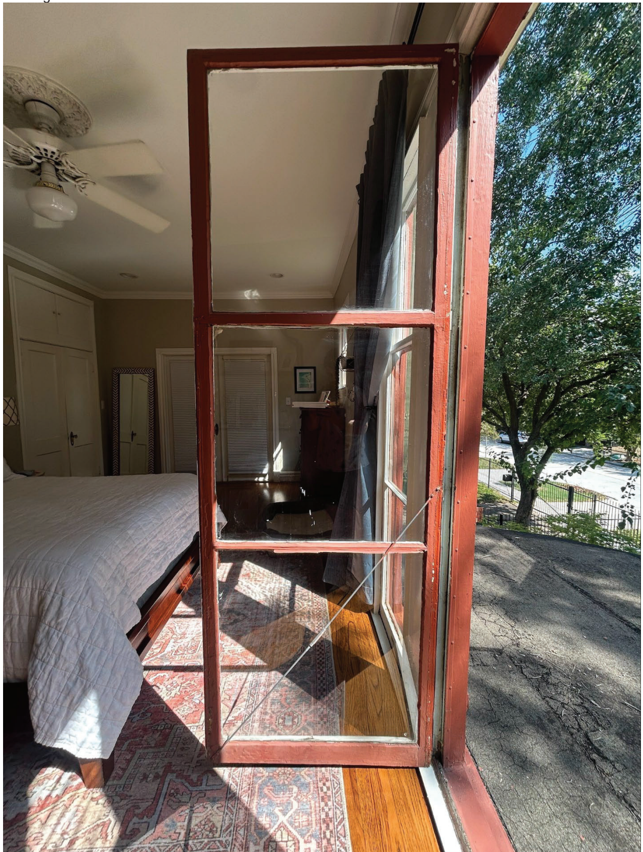
Existing window converted into door
