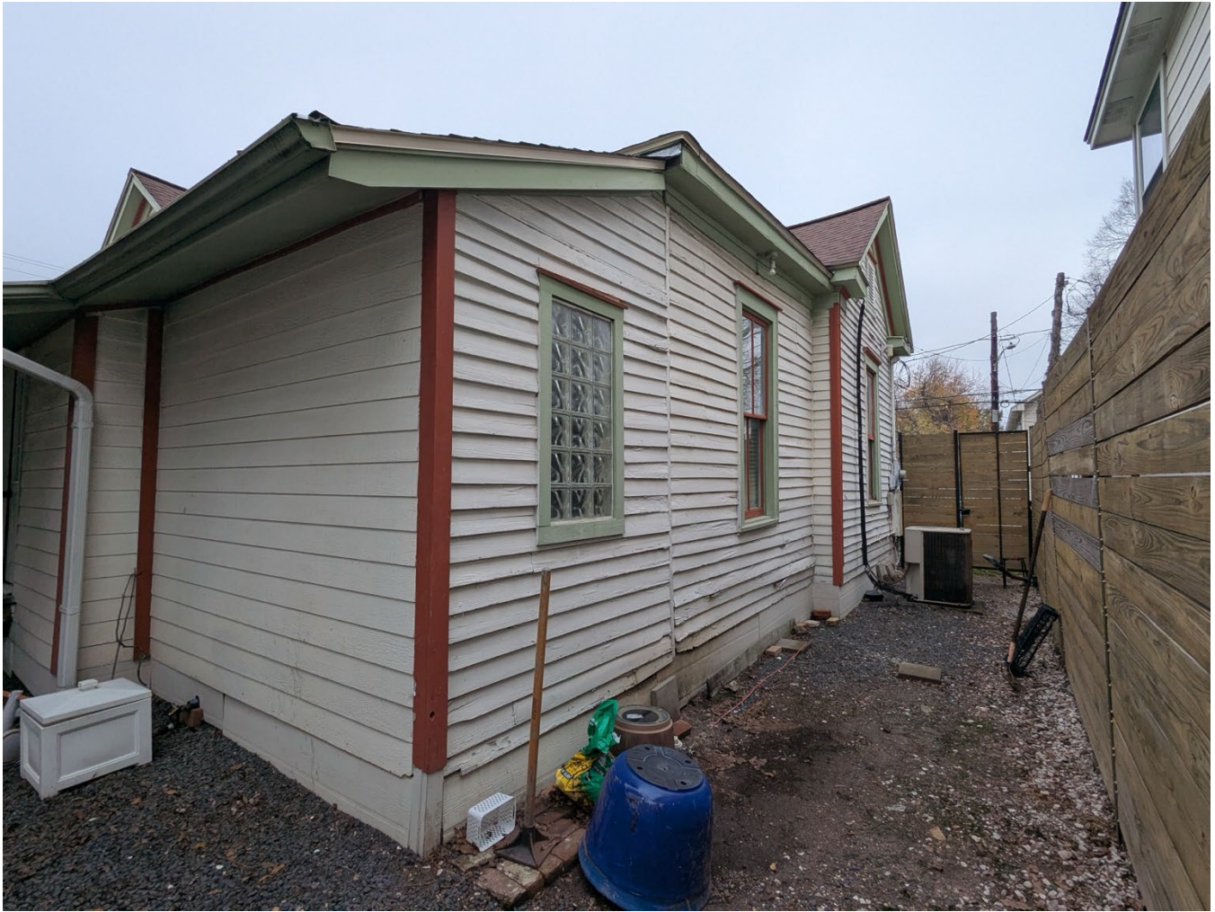
SOUTHEAST CORNER, FACING NORTHWEST
