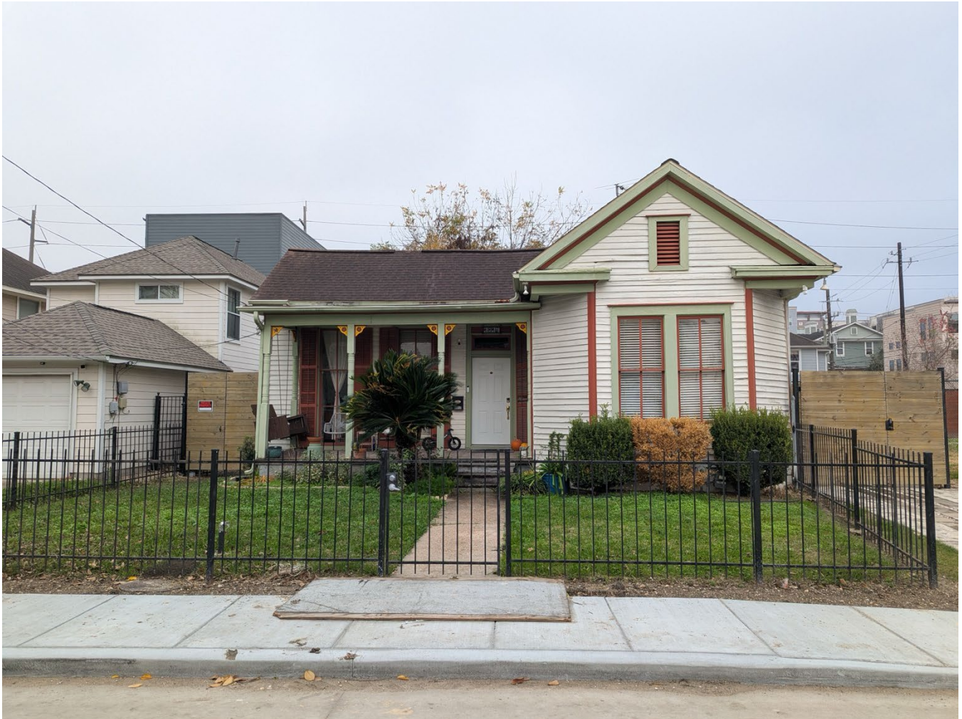
FRONT ELEVATION, FACING SOUTH
