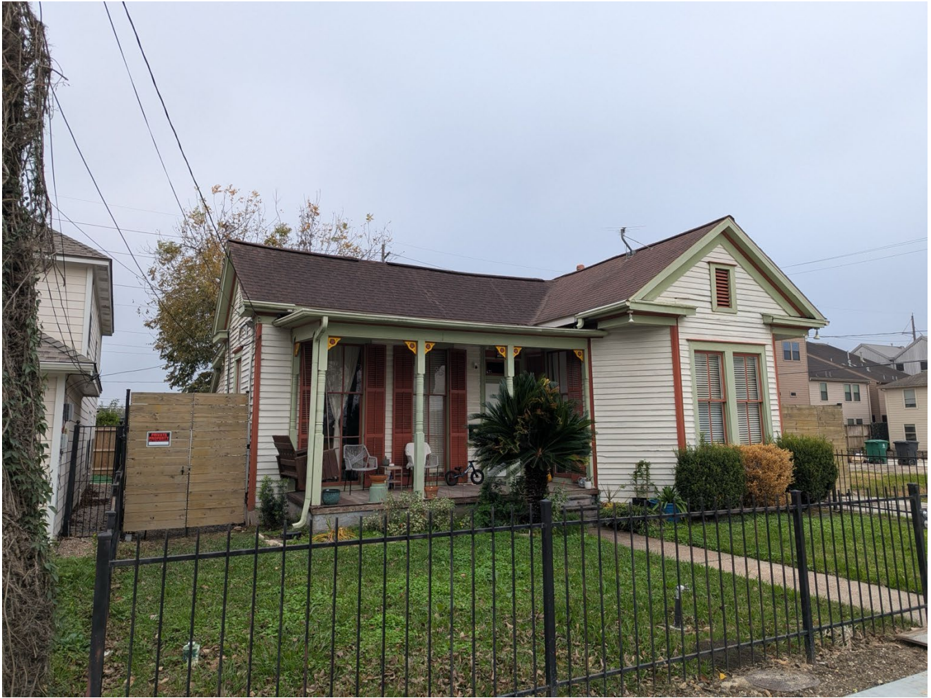
NORTHEAST CORNER, FACING SOUTHWEST
