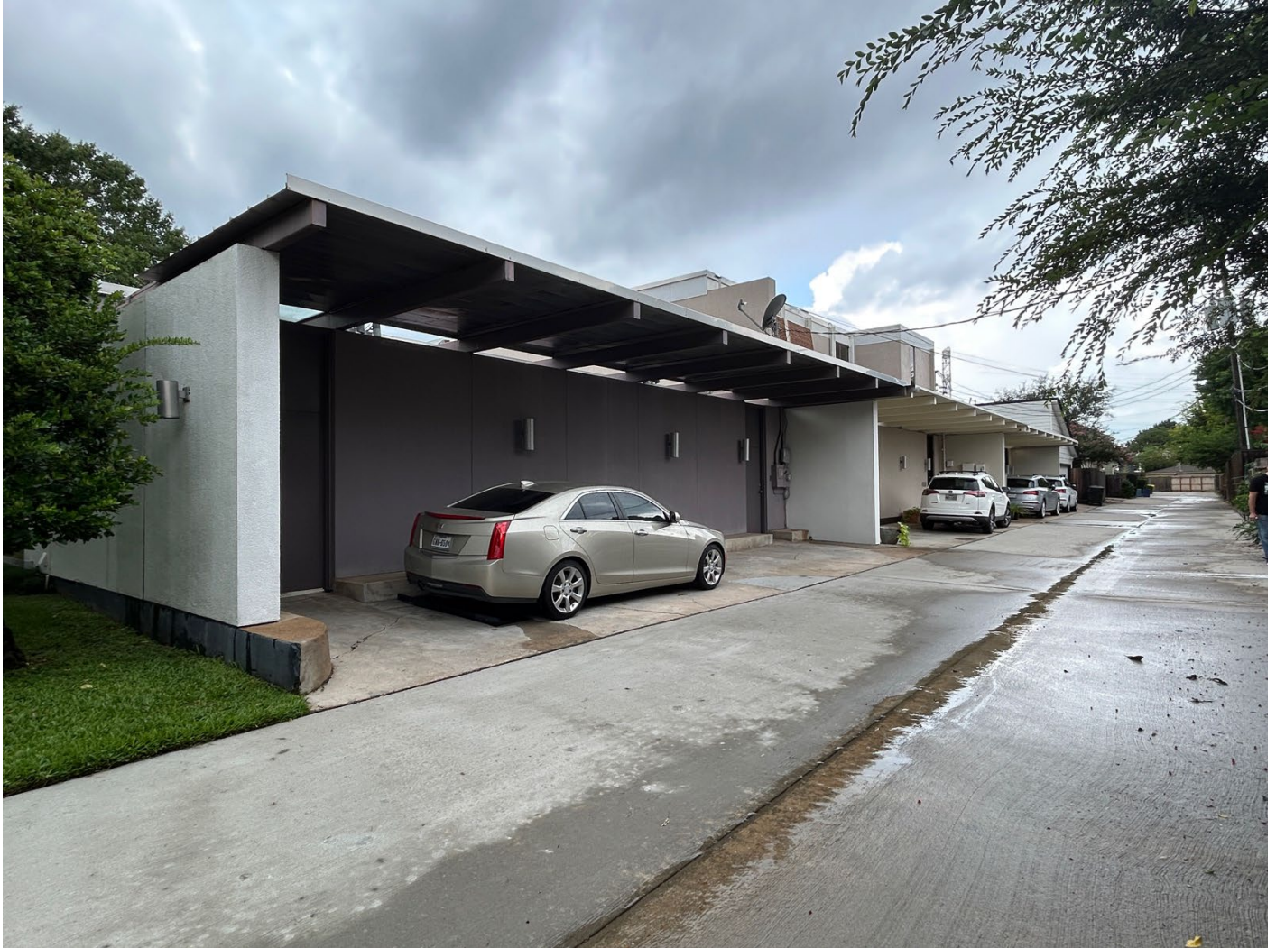
Photo 6. All three townhouses, oblique view of carports and alley, camera facing west.
