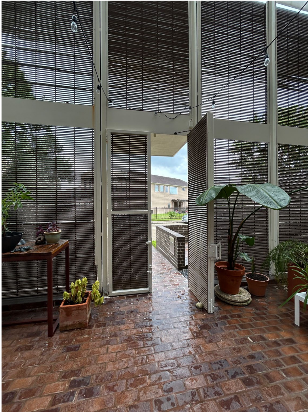
Photo 23. Unit B, front courtyard gate and louvered screens, camera facing south.
