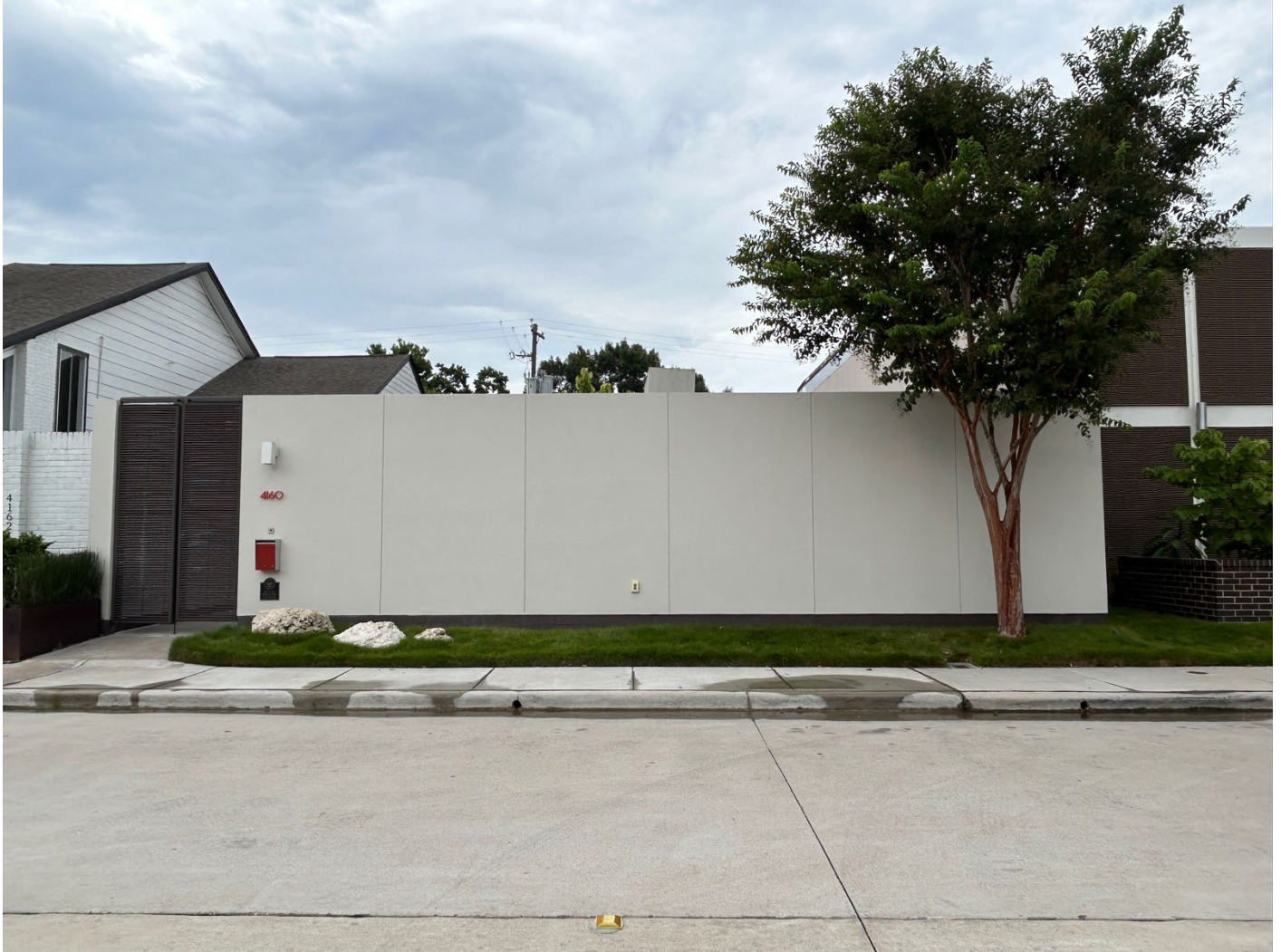
Photo 2. Unit A/4160 Meyerwood, front (south) elevation, camera facing north.
