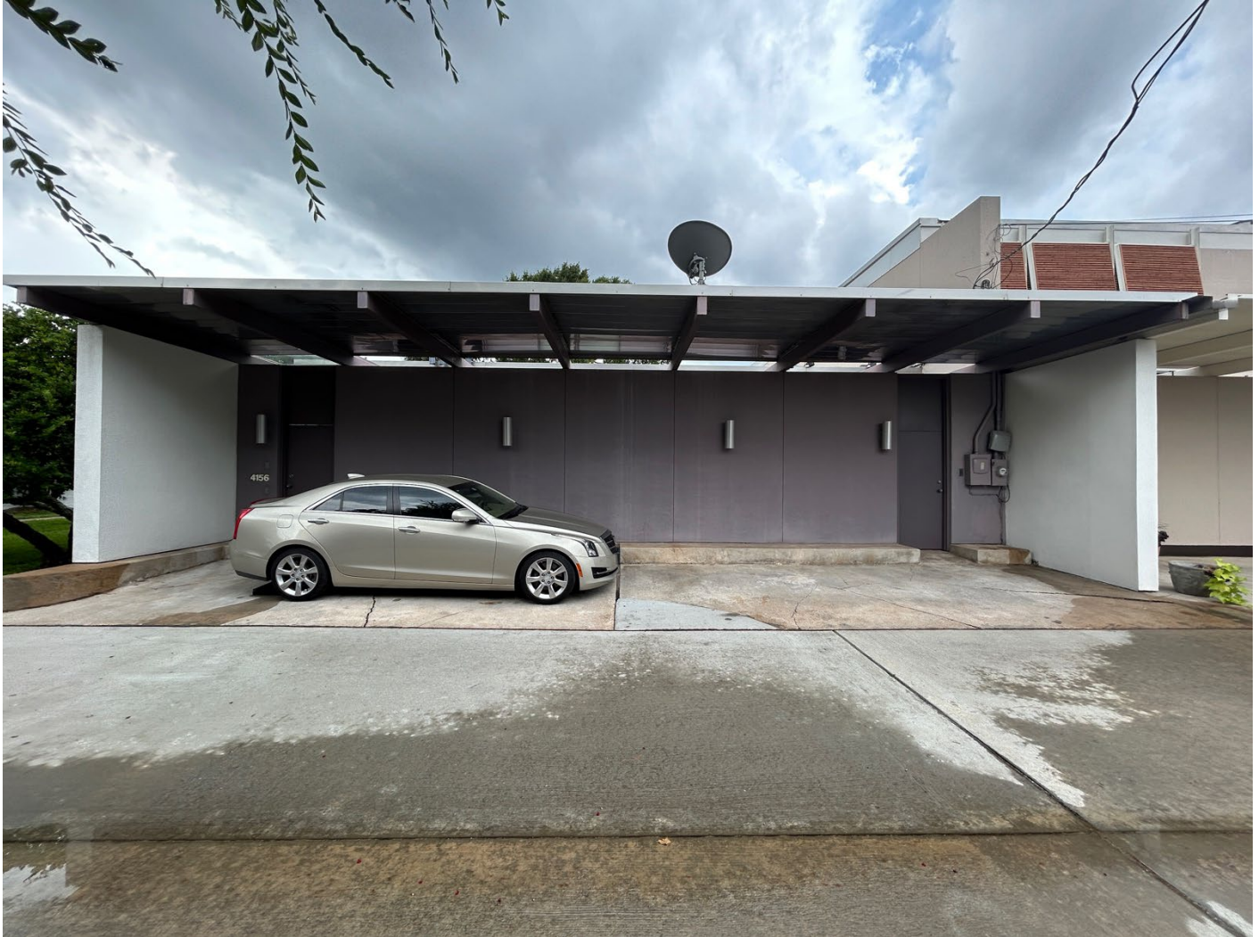
Photo 7. Unit C, carport, camera facing south.
