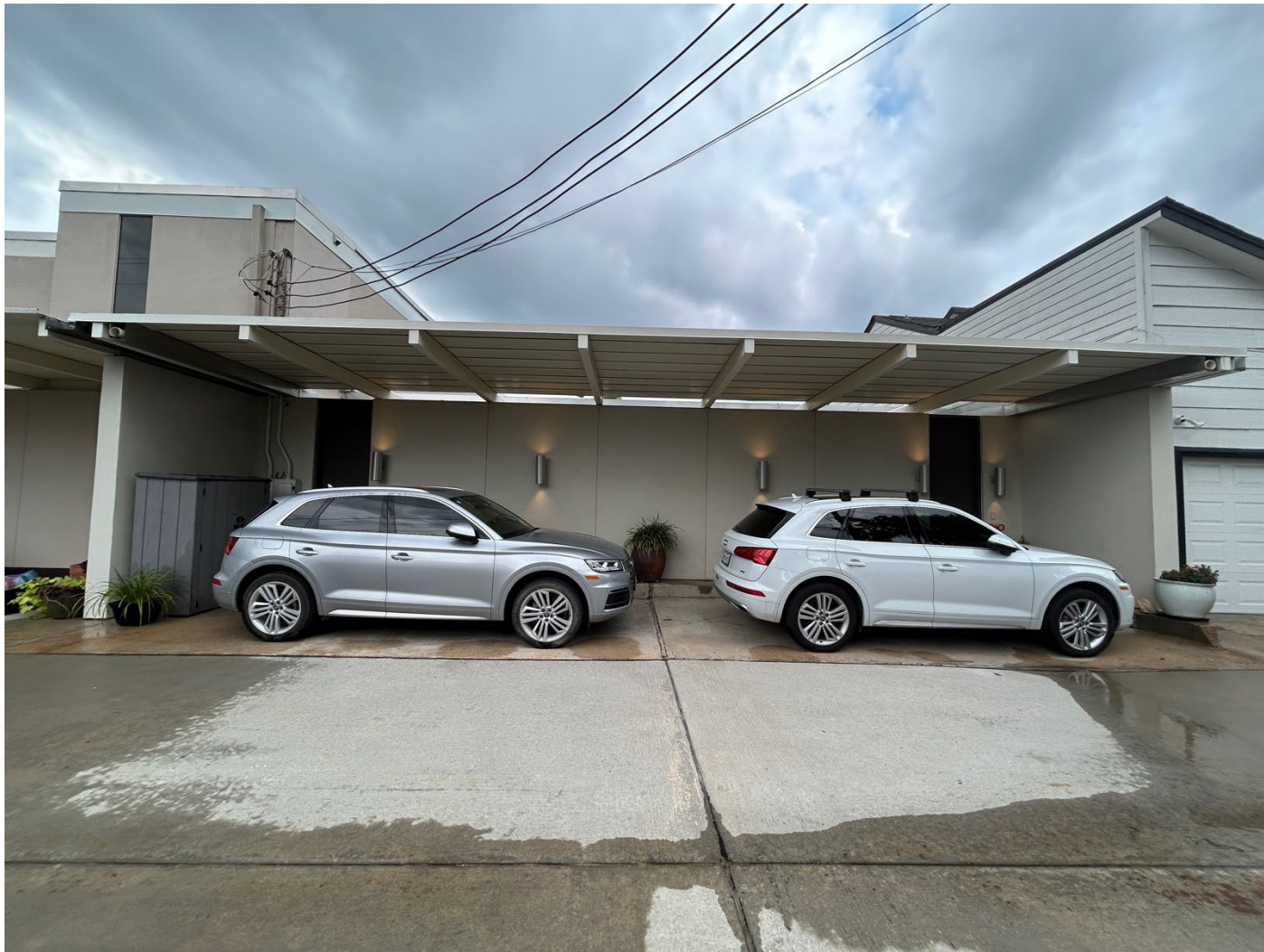
Photo 9. Unit A, carport, camera facing south.
