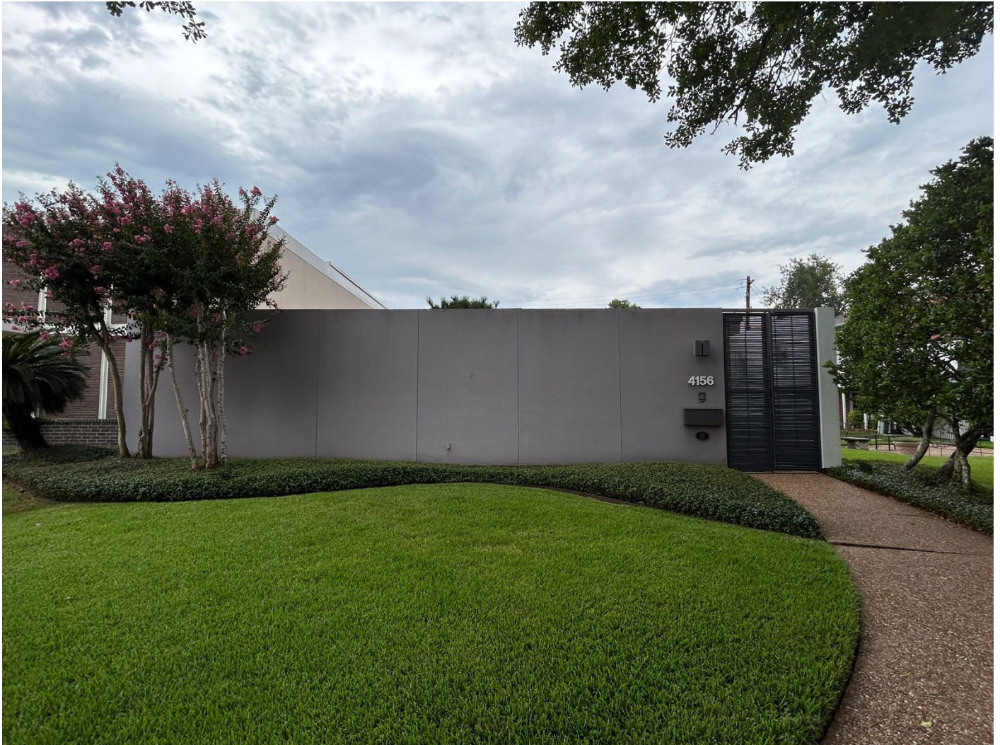
Photo 4. Unit C/4156 Meyerwood, front (south) elevation, camera facing north.
