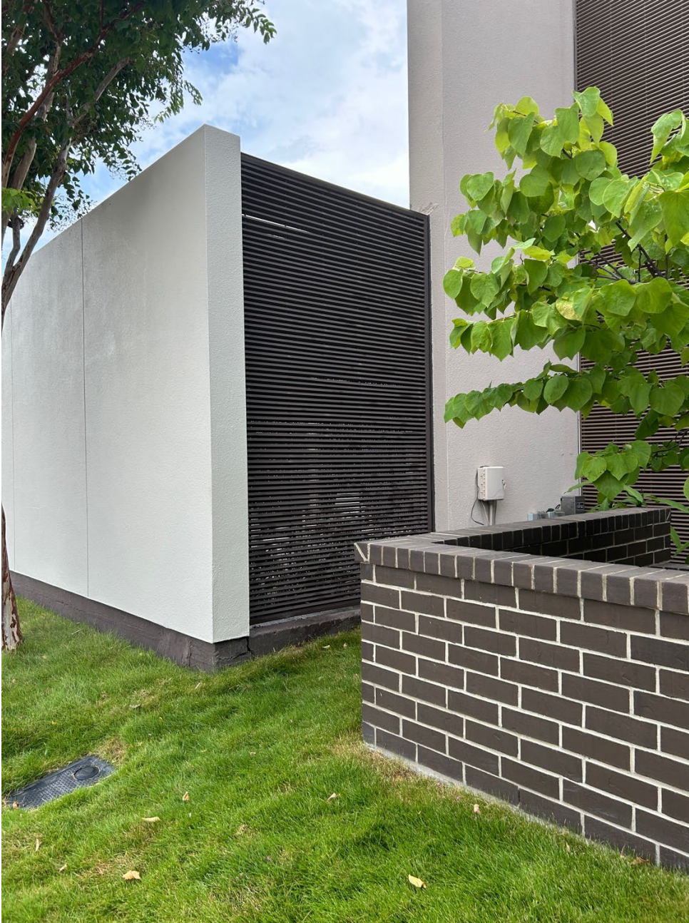
Photo 11. Unit A, screen panel in eastern courtyard wall, camera facing northwest.
