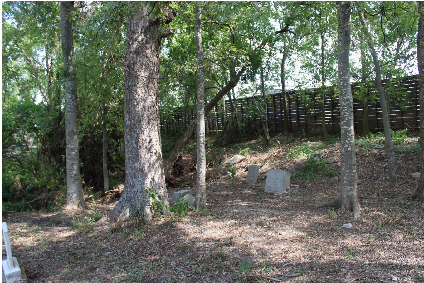
Photo 8. Gully erosion, camera facing northeast
