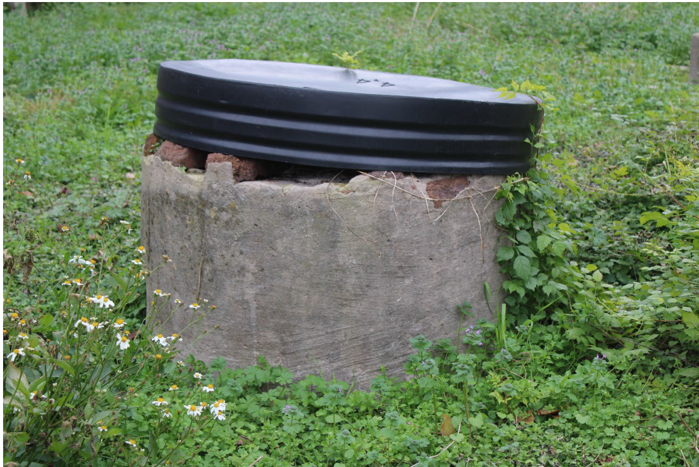
Photo 40. Concrete and brick well or cistern, camera facing southeast
