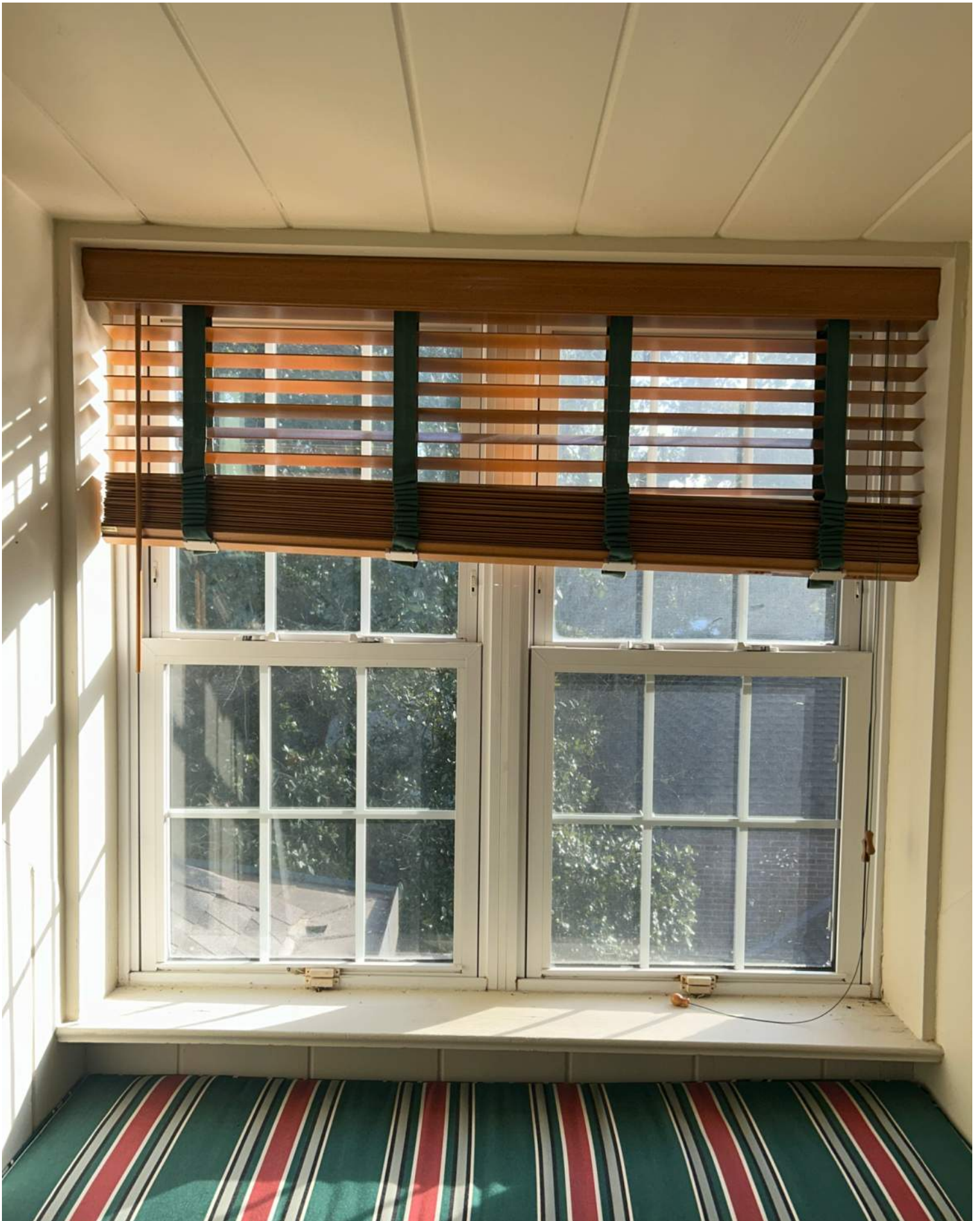
W14.2 (Existing Third Floor Dormer Window)
