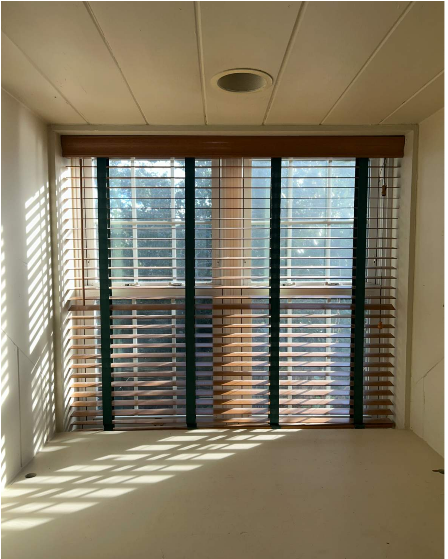
W14.1(Existing Third Floor Dormer Window)
