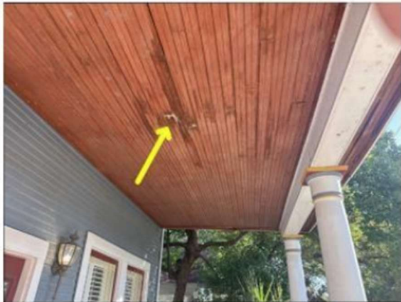
Water stains, observed below balcony
