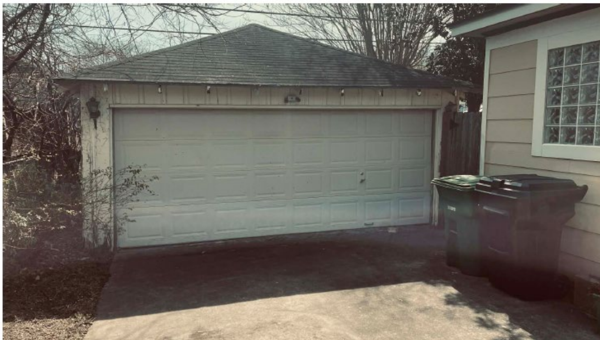
North elevation of garage.
