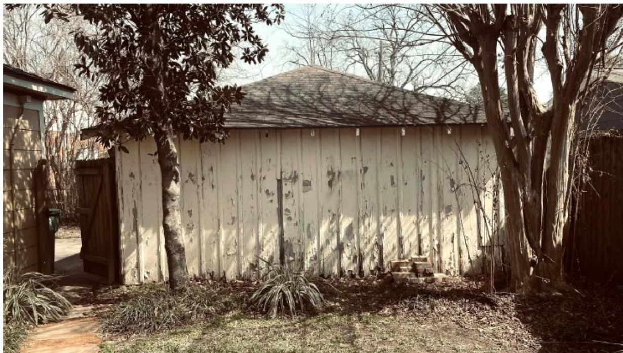
West elevation of garage.
