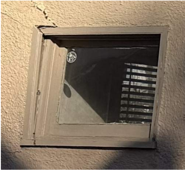
SIDE (WEST ELEVATION) #19 TO BE REPLACED WITH NEW TO MATCH EXISTING
