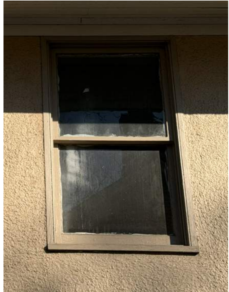
SIDE (WEST ELEVATION) #25 TO BE REPLACED WITH NEW TO MATCH EXISTING
