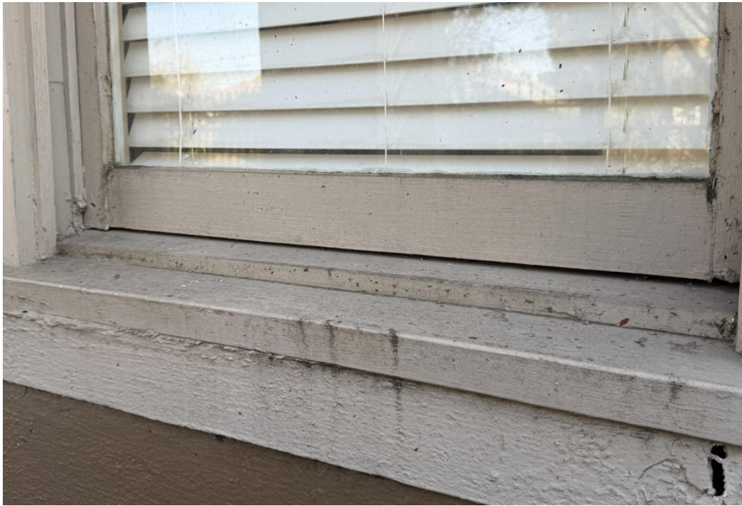
EXISTING 503 SUL ROSS SINGLE HUNG WOOD WINDOW WITH WINDOW STOOL
