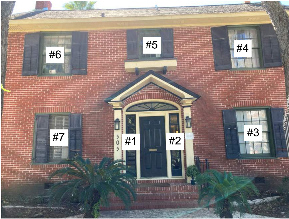
505 SUL ROSS - FRONT (NORTH ELEVATION)
