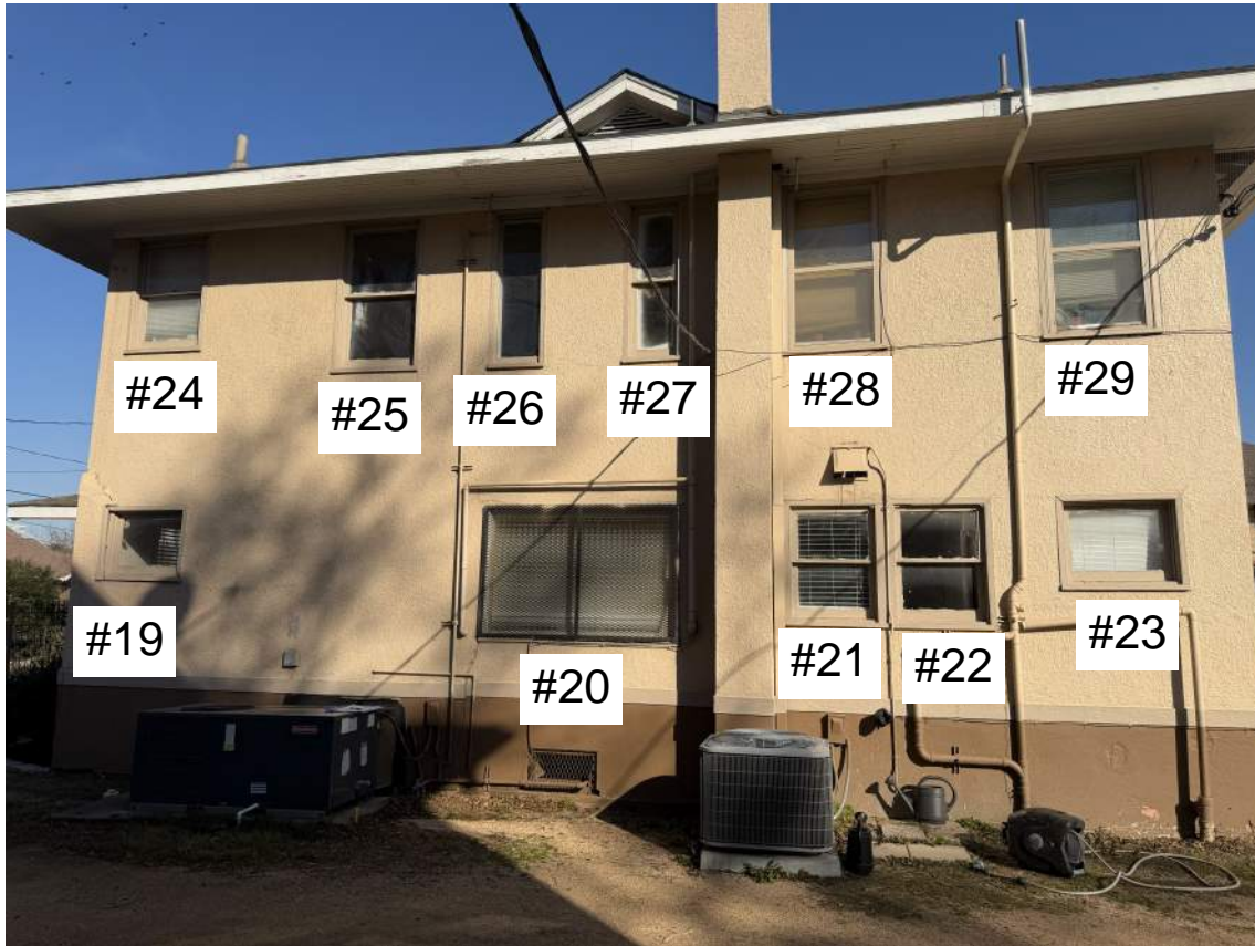
503 SUL ROSS - SIDE (WEST ELEVATION)
