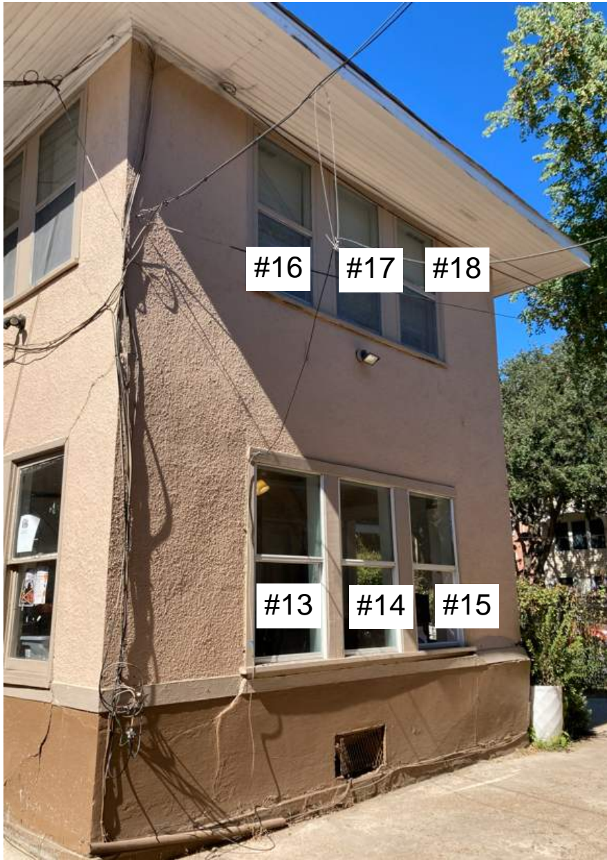
503 SUL ROSS - SIDE (EAST ELEVATION)
