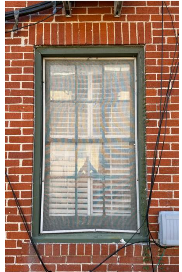
SIDE (EAST ELEVATION) #12 TO BE REMOVED, REFER TO ORIGINAL COA APPLICATION, CONFLICT WITH WALL
