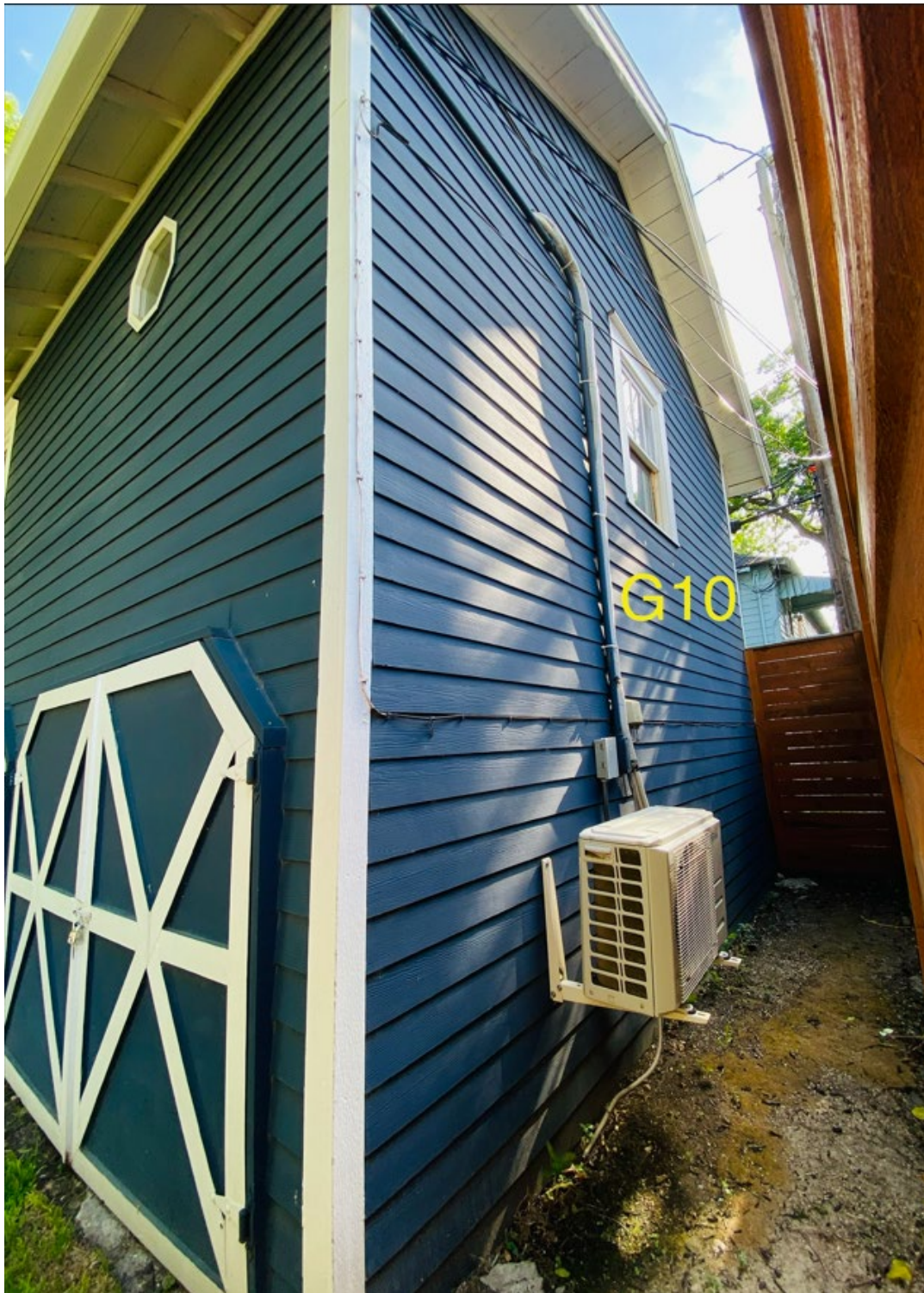
CURRENT PHOTO – GARAGE AT REAR (NON-CONTRIBUTING)
