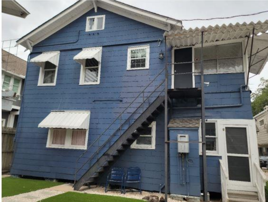
Back Side of Front Building
