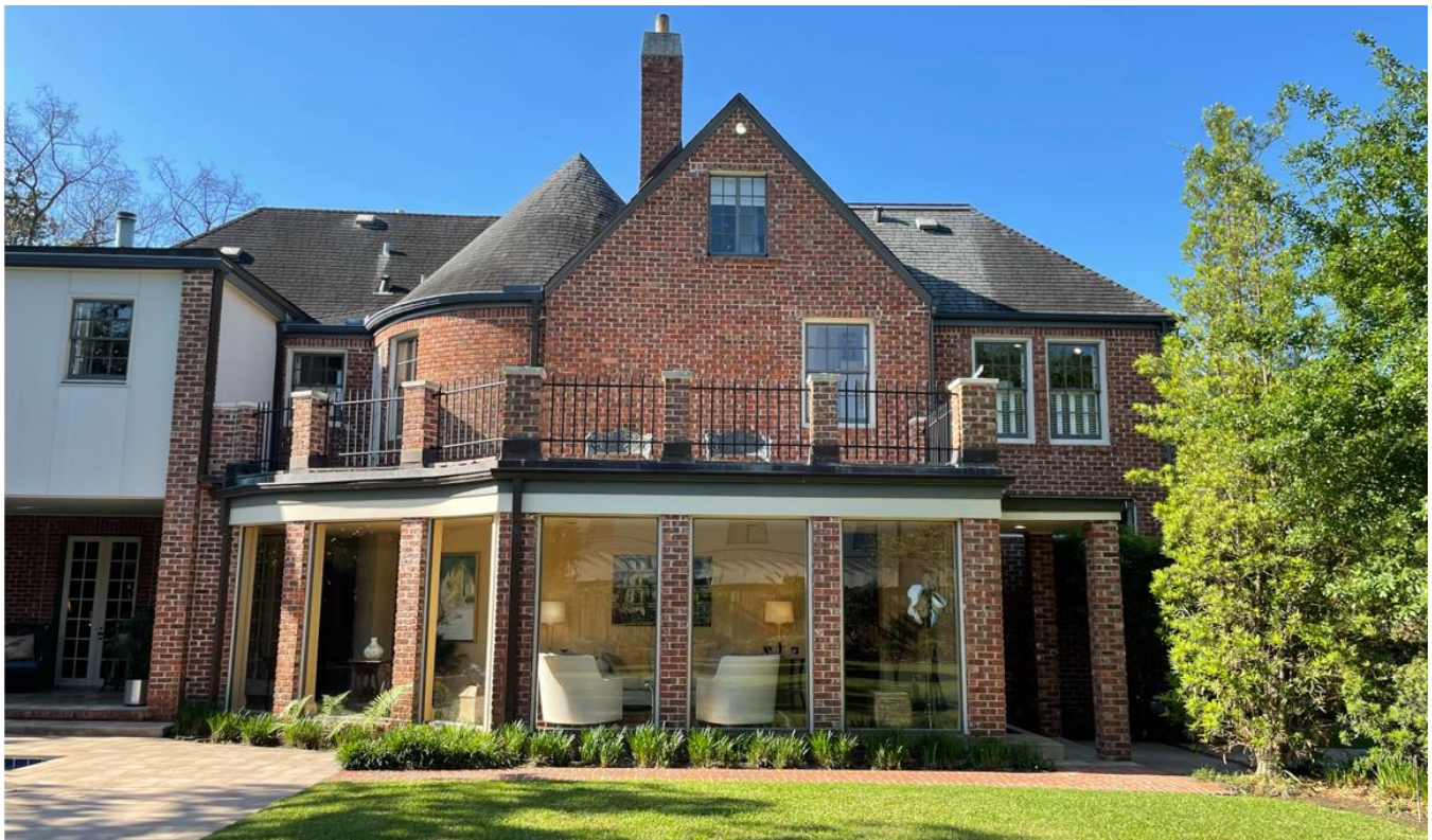
Porch enclosed/alterd after c. 1980
