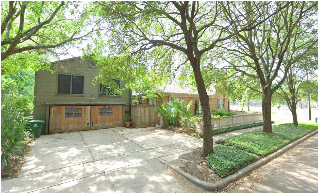
Figure 4 - Looking NW at garage apt and house
