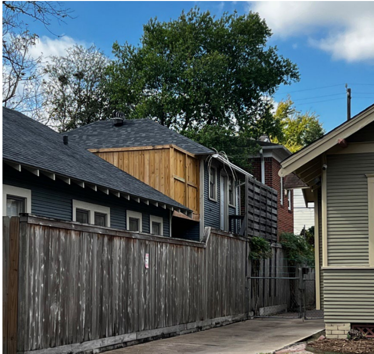
Figure 2- Side north elevation showing Privacy wall covering second story porch
