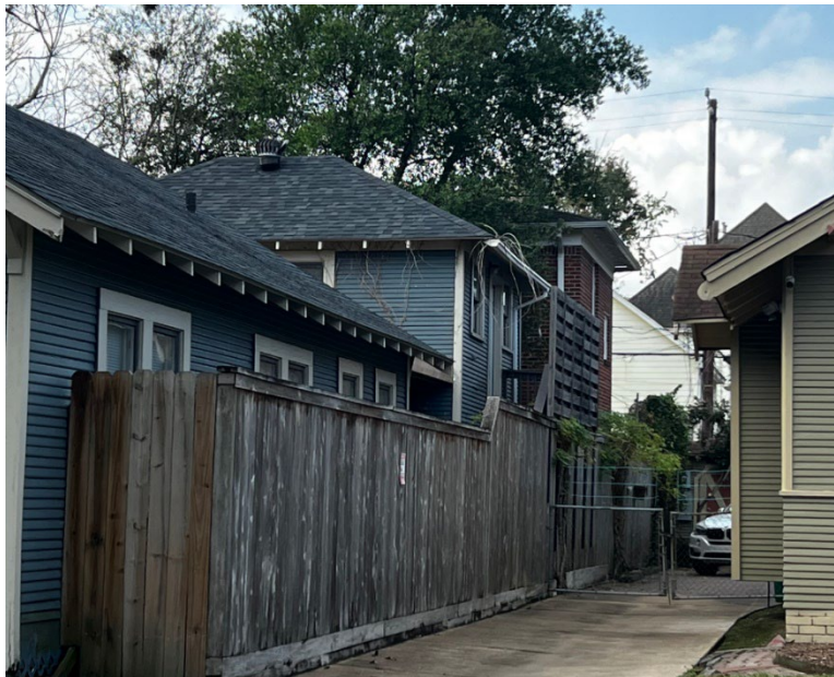
Figure 1- Side north elevation _ Privacy wall removed
