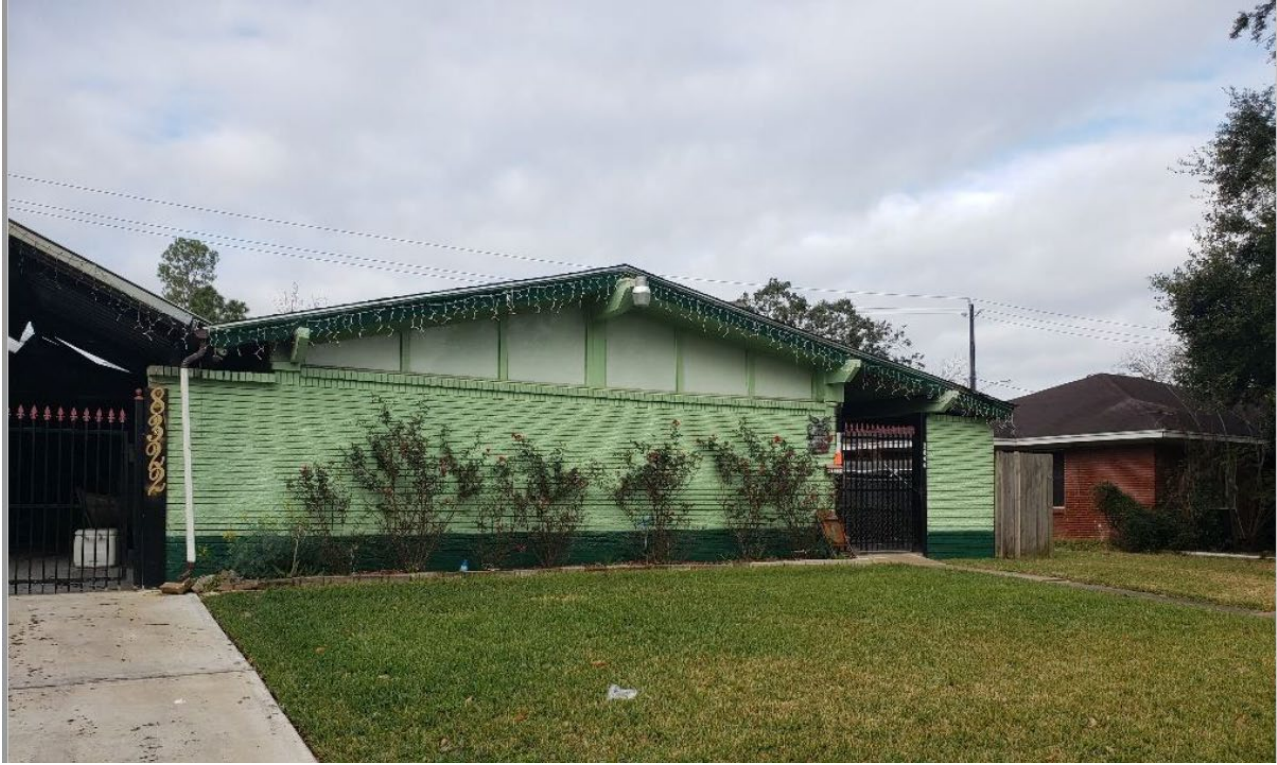
Figure 8 - 1/26/22 After the Fire - Facade Intact from Violation Notice
