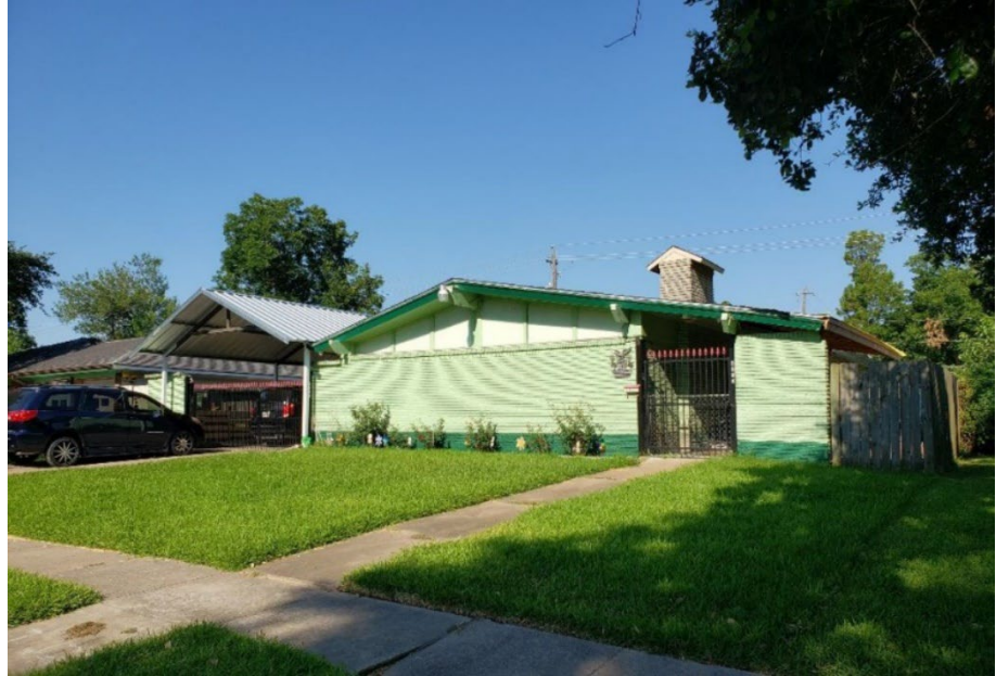
Figure 3 - 6/16/2020 First Violation Notice
