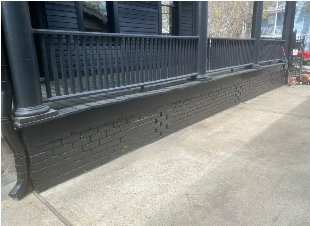
(Side elevation visible from the street)
