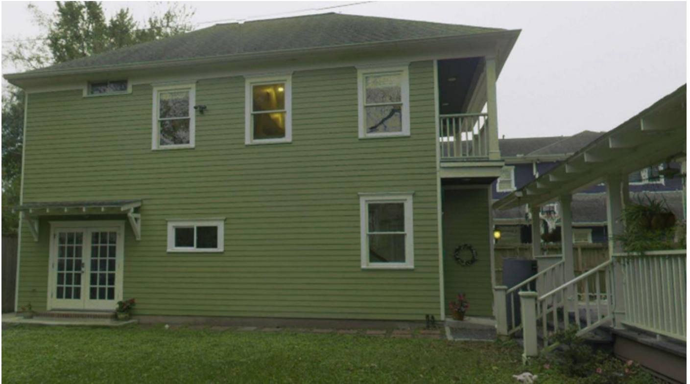
Photograph of North Elevation of Garage/ East Elevation of House
