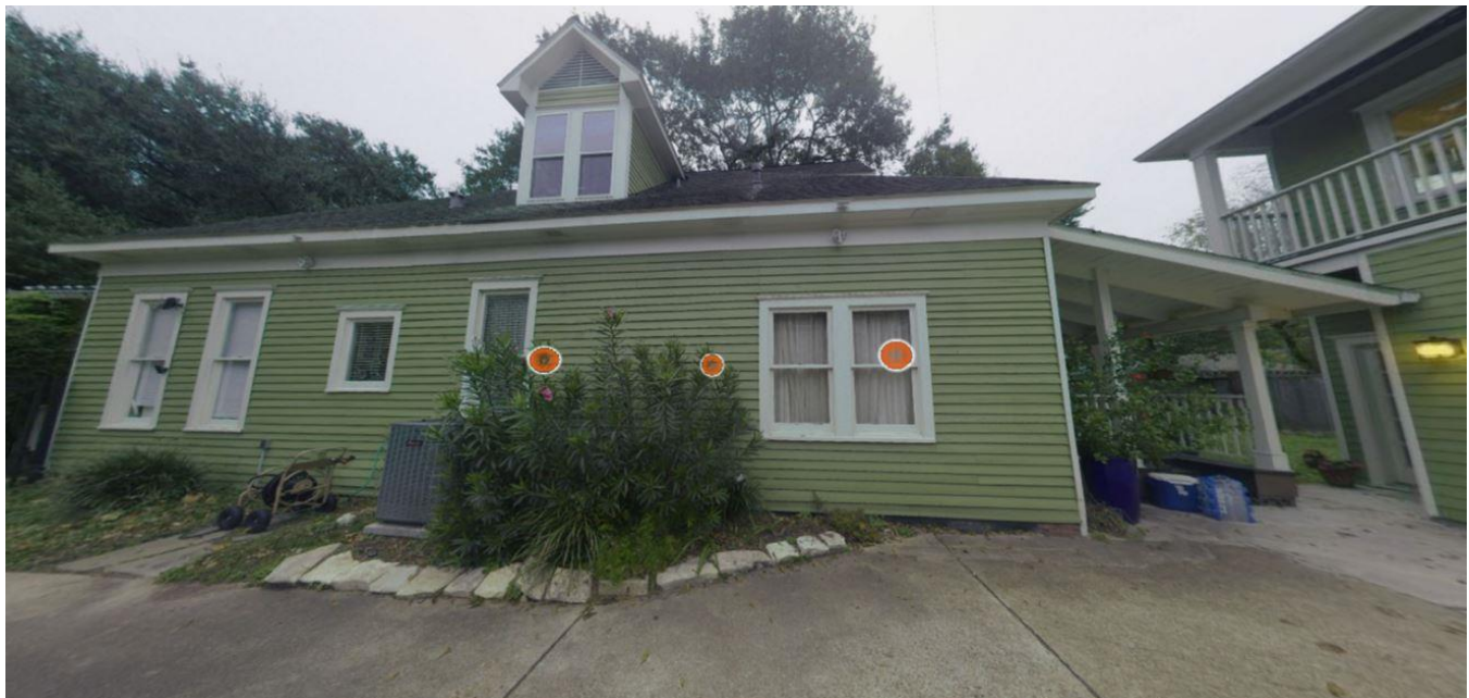
Photograph of South Elevation (Right)
