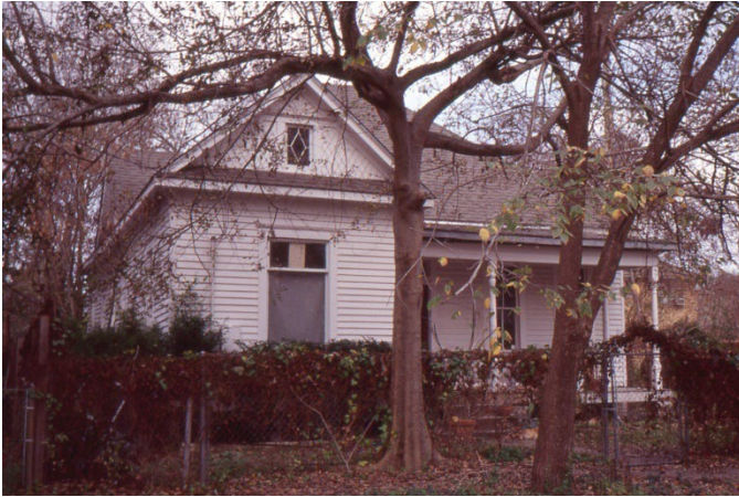
Figure 1_2014 State St. _next door neighbor
