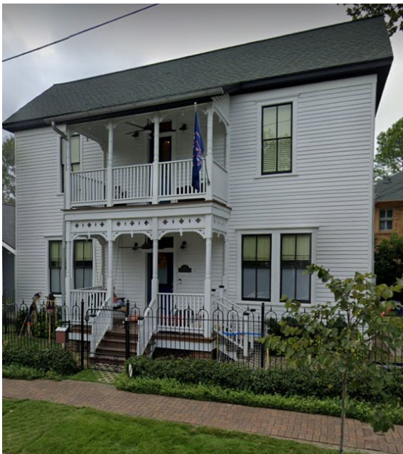
Figure 1_609 White St._ example of contributing tall structures in the context area
