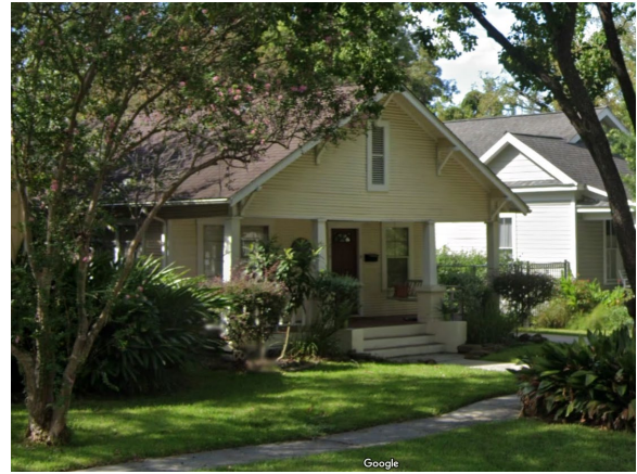
1219 Oxford – Contributing – (neighboring)
