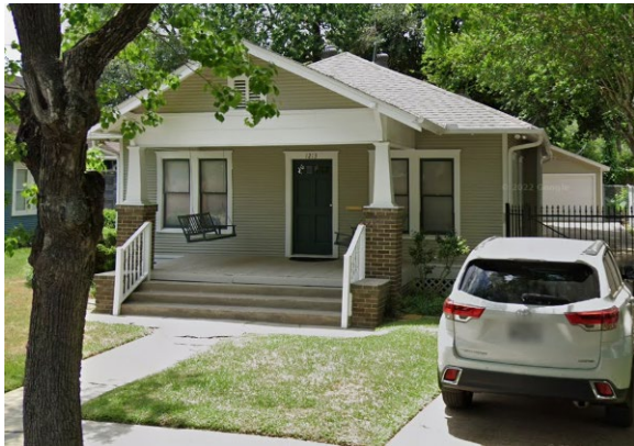
1213 Oxford – Contributing – (neighboring)
