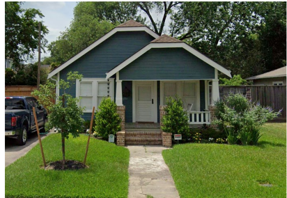
1209 Oxford – Contributing – 1915 (neighboring)
