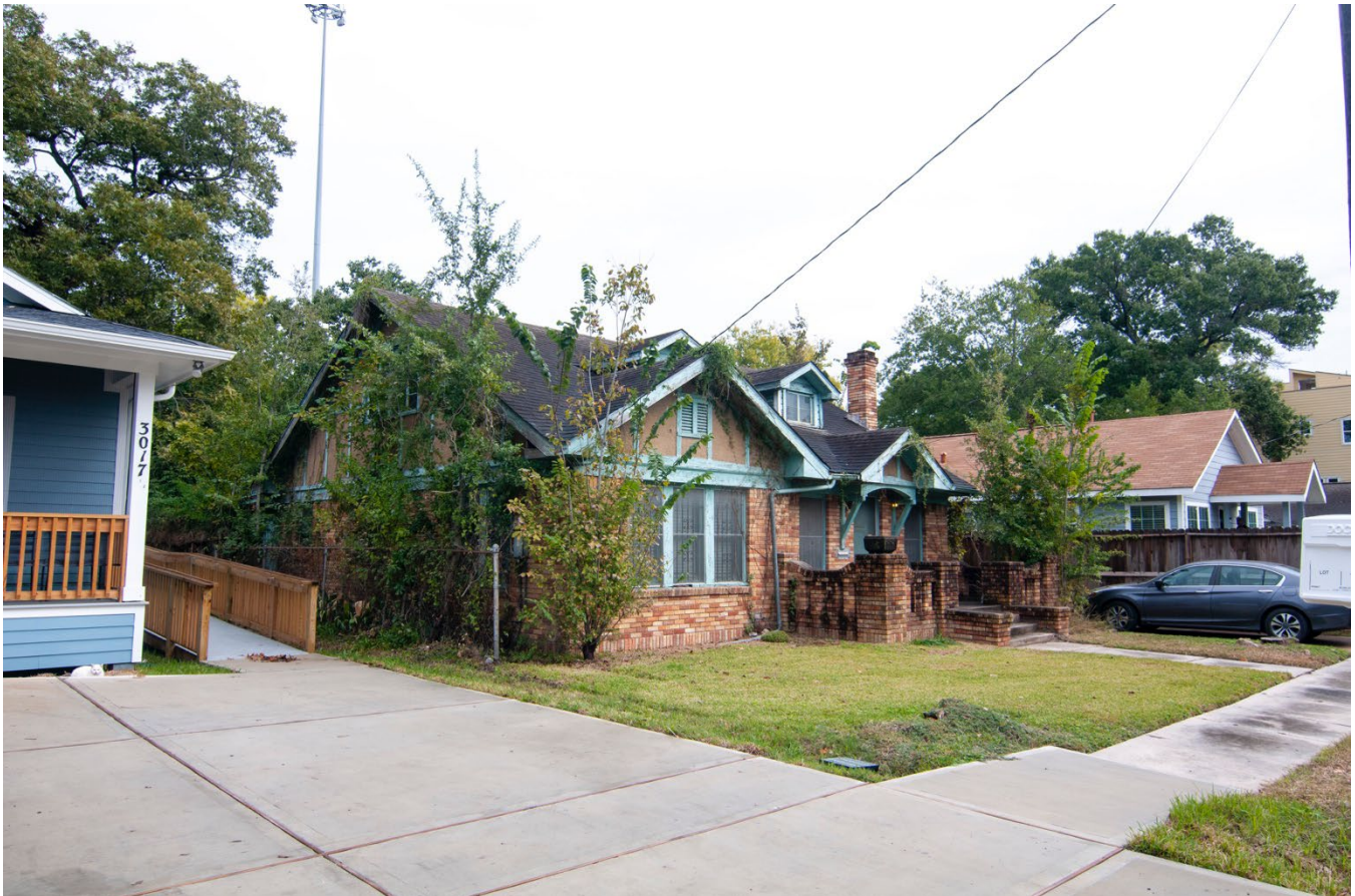
Southwest corner and adjacent buildings, facing east
