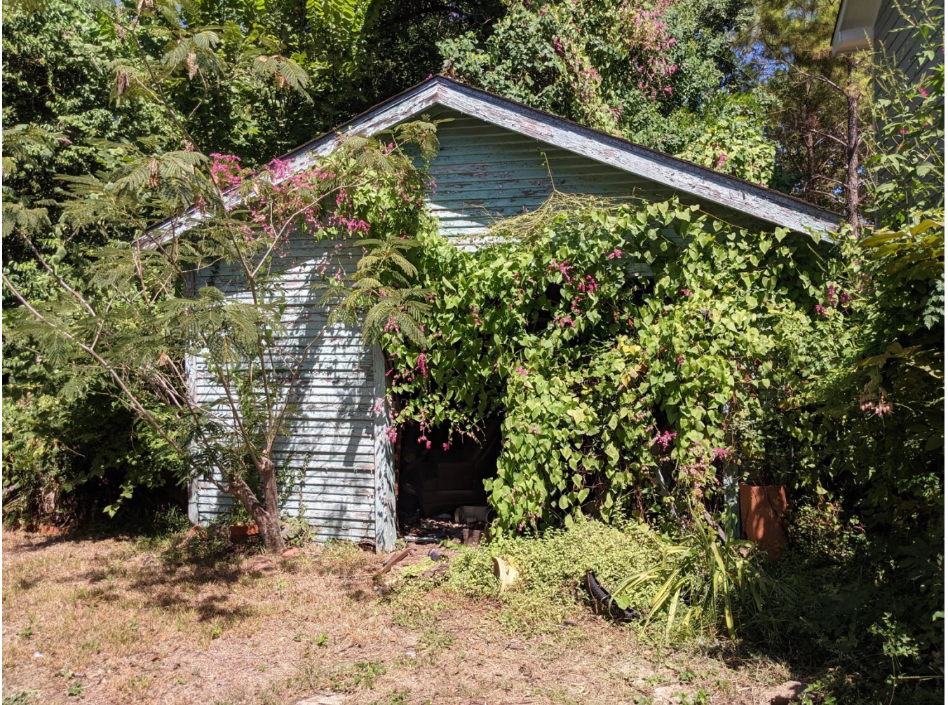
Garage, facing northeast
