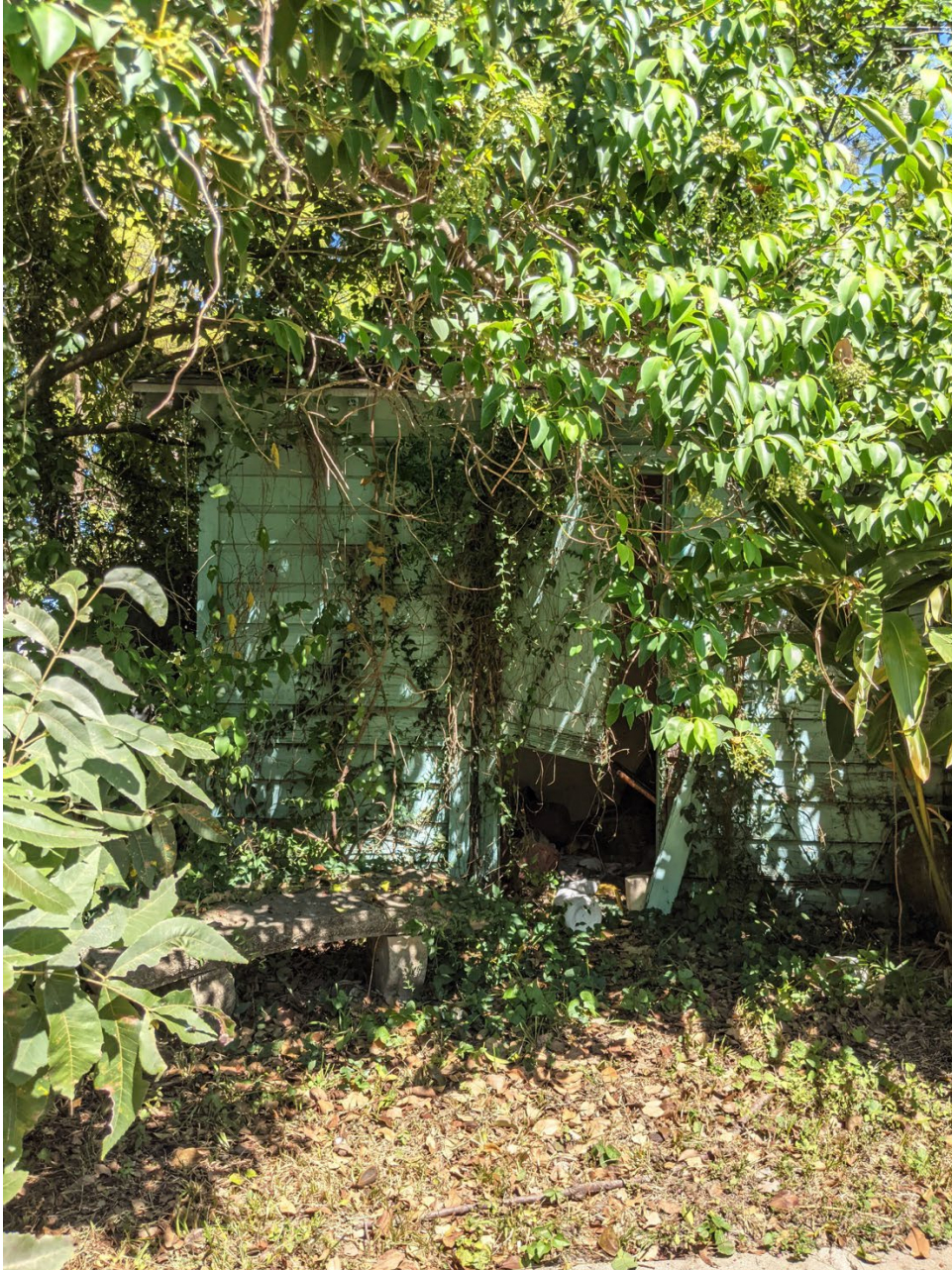
Shed, facing northeast
