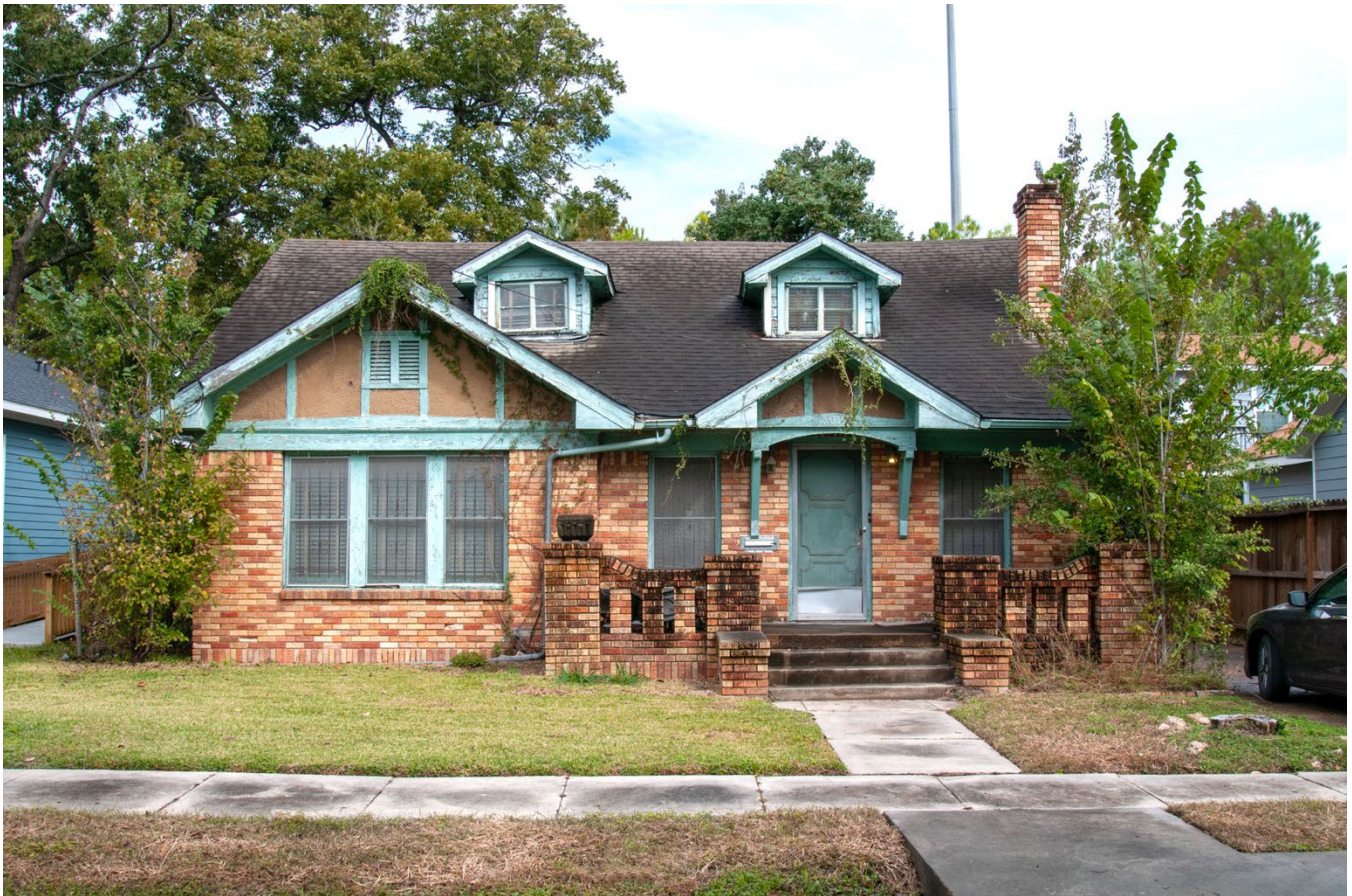
Southwest (front) elevation, facing northeast
