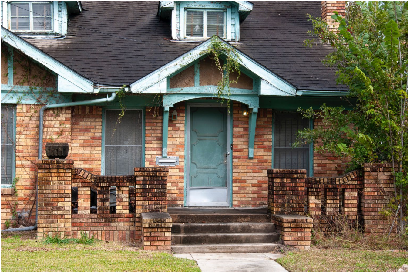
Terrace and entrance, facing northeast
