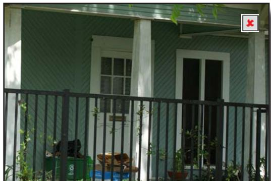
*Siding applied in an incompatible herringbone pattern*
