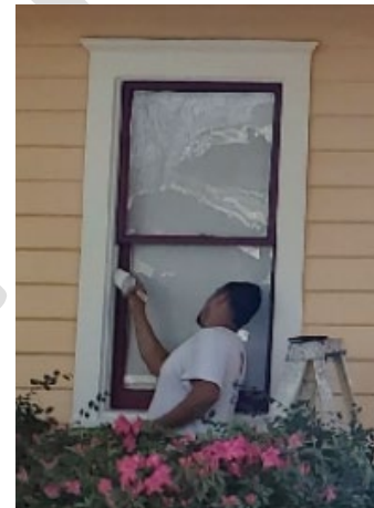
Historic materials should maintain protective coatings such as paint to prolong the life of the material.
