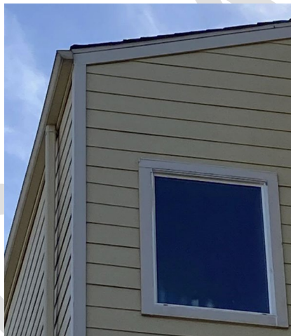
Do not cut back a roof eave so it is flush with the wall.
