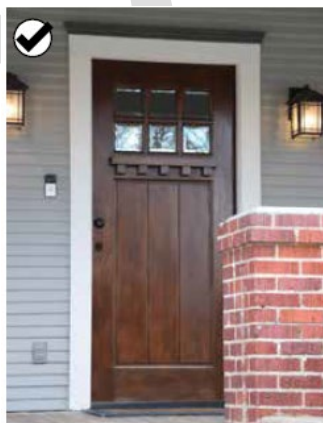
If a door cannot be repaired, match its replacement to the original.
