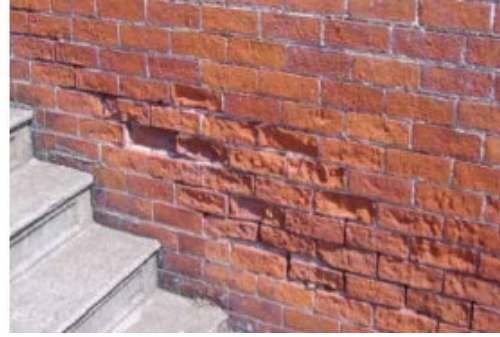
Brick showing damage from inappropriate cleaning (photo courtesy of Heritage Ohio).
