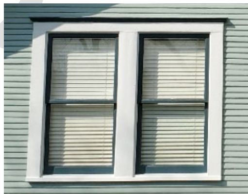
Example of intact historic one-over-one wood windows.
