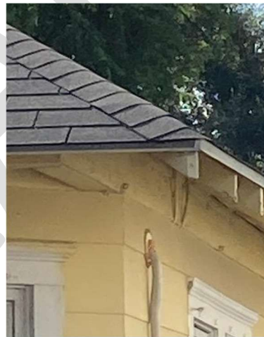
Preserve the original eave depth and design. While the eave depth and design are intact, the building is still in need of some maintenance to protect these features.
