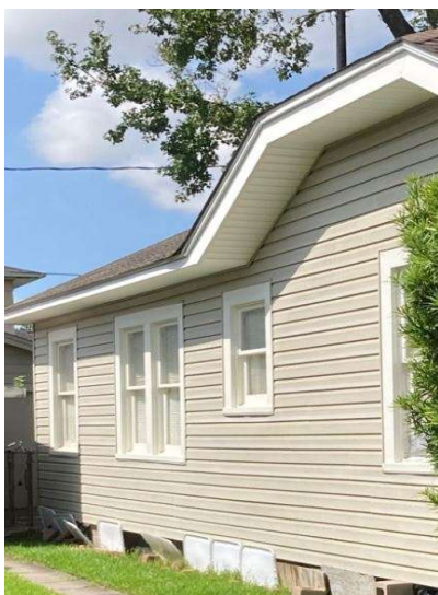
Typical siding profiles in Norhill: (left) 105 and (right) 117. The most common type of siding found on historic houses in the Norhill Historic District is wood siding.
