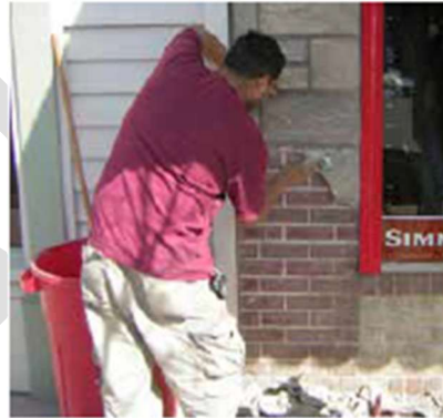
Consider removing later covering materials that have not achieved historic significance. Once the non-historic siding is removed, repair the original underlying material.
