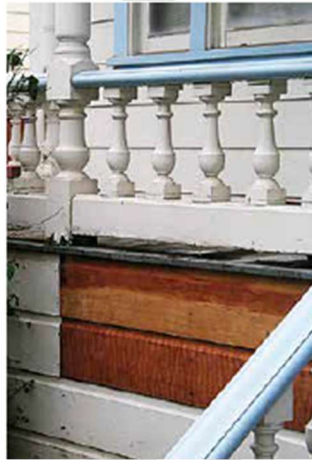
If repair is not possible, replace only the damaged wood.
