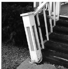
(Left) Before Repair: A deteriorated post and handrail.
